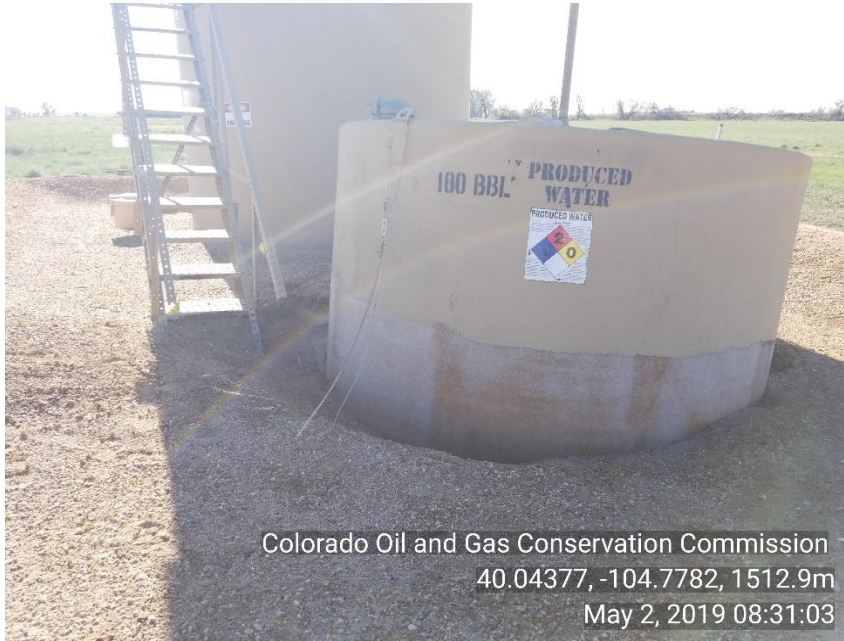
Photo 3 Produced water tank appears to have floated out of ground.
