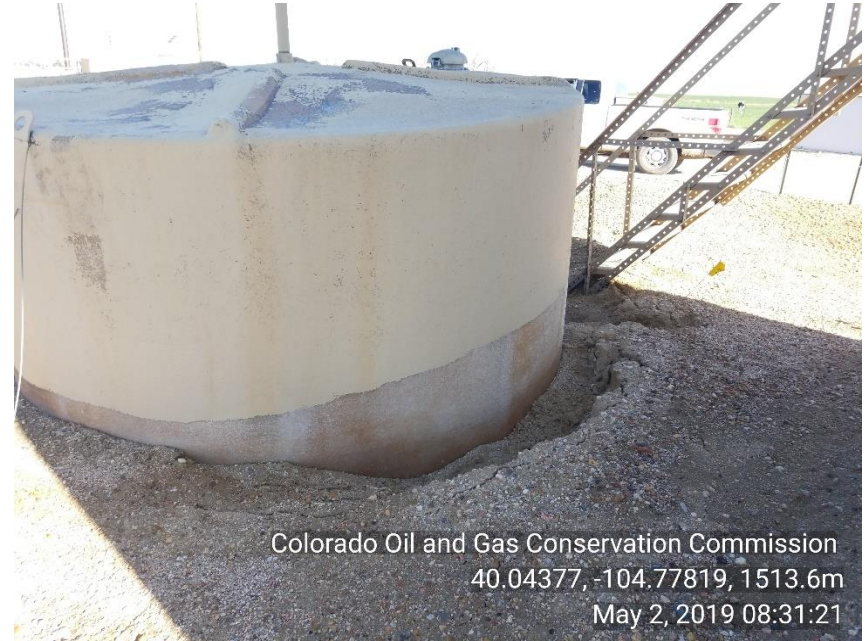
Photo 4 Produced water tank appears to have floated out of ground. Possible under ground issues.
