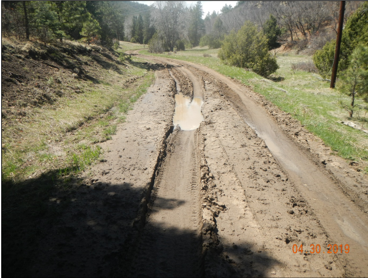
Photo 2. There are deep vehicle ruts along the road. Stormwater is accumulating on the road.
