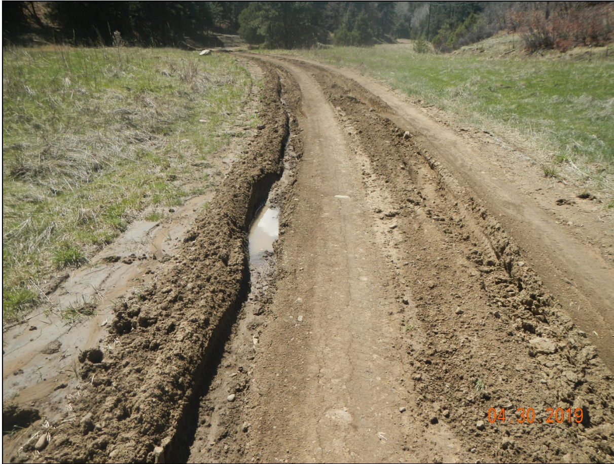
Photo 1. Facing west along the main access road. There is vehicle rutting along the road causing road damage.
