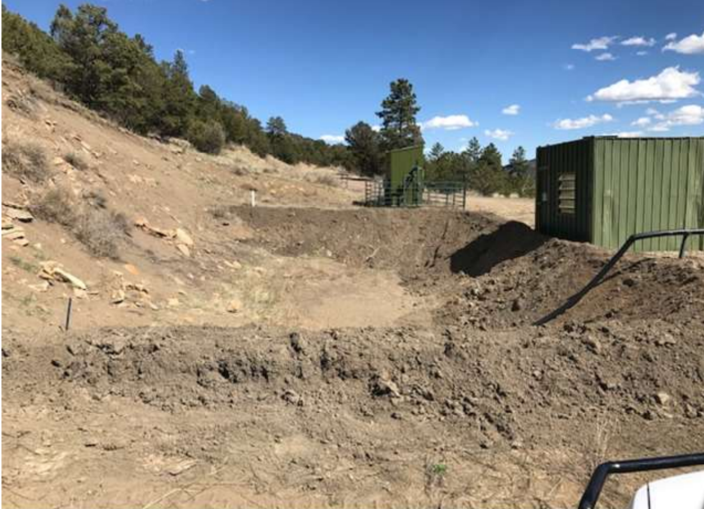
PHOTO 3: A DIRT BERM WAS ESTABLISHED AROUND THE PRODUCTION PIT.
