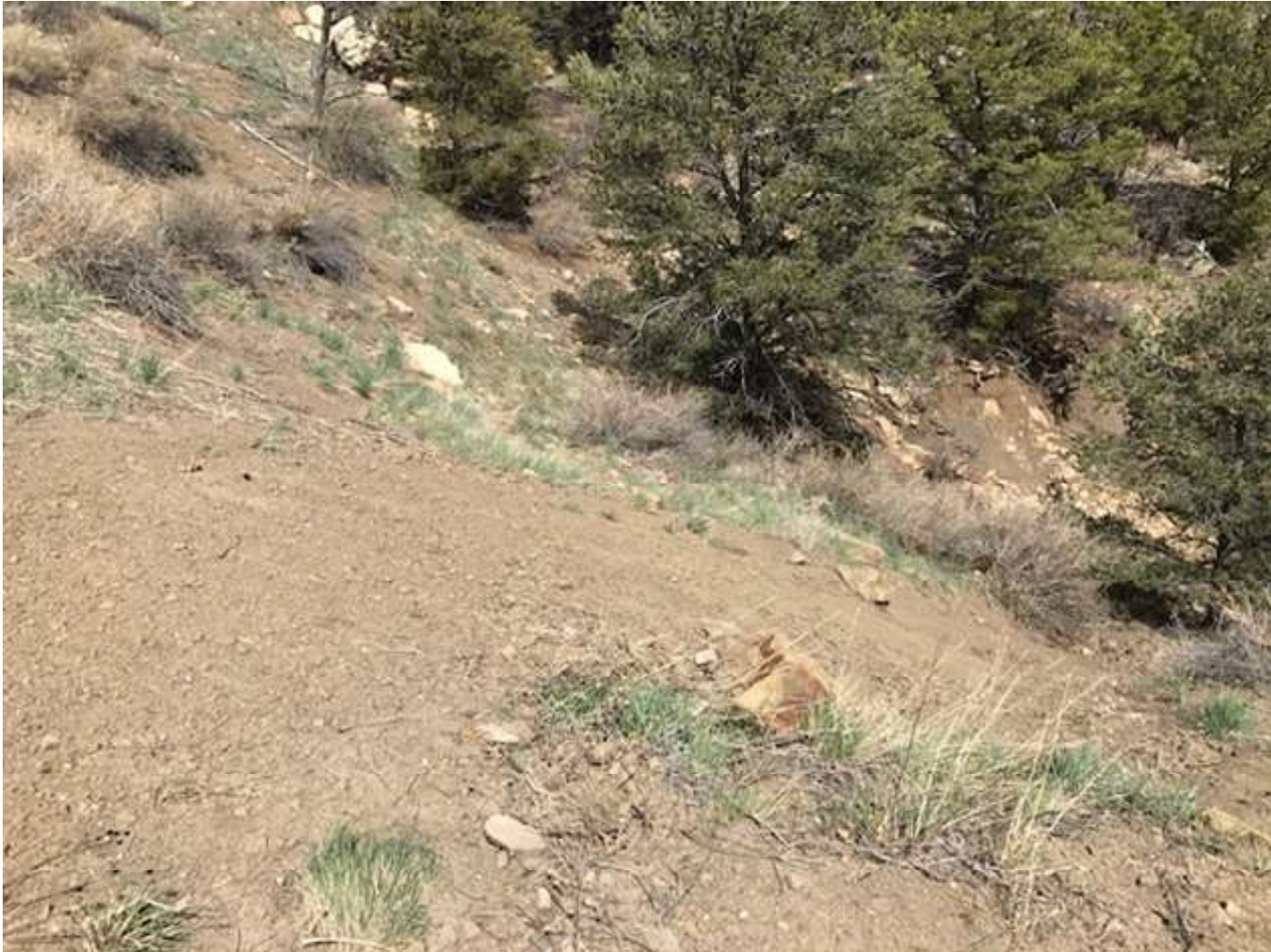
PHOTO 5: THE EROSION RILL ON THE FILL SLOPE WAS FILLED IN.
