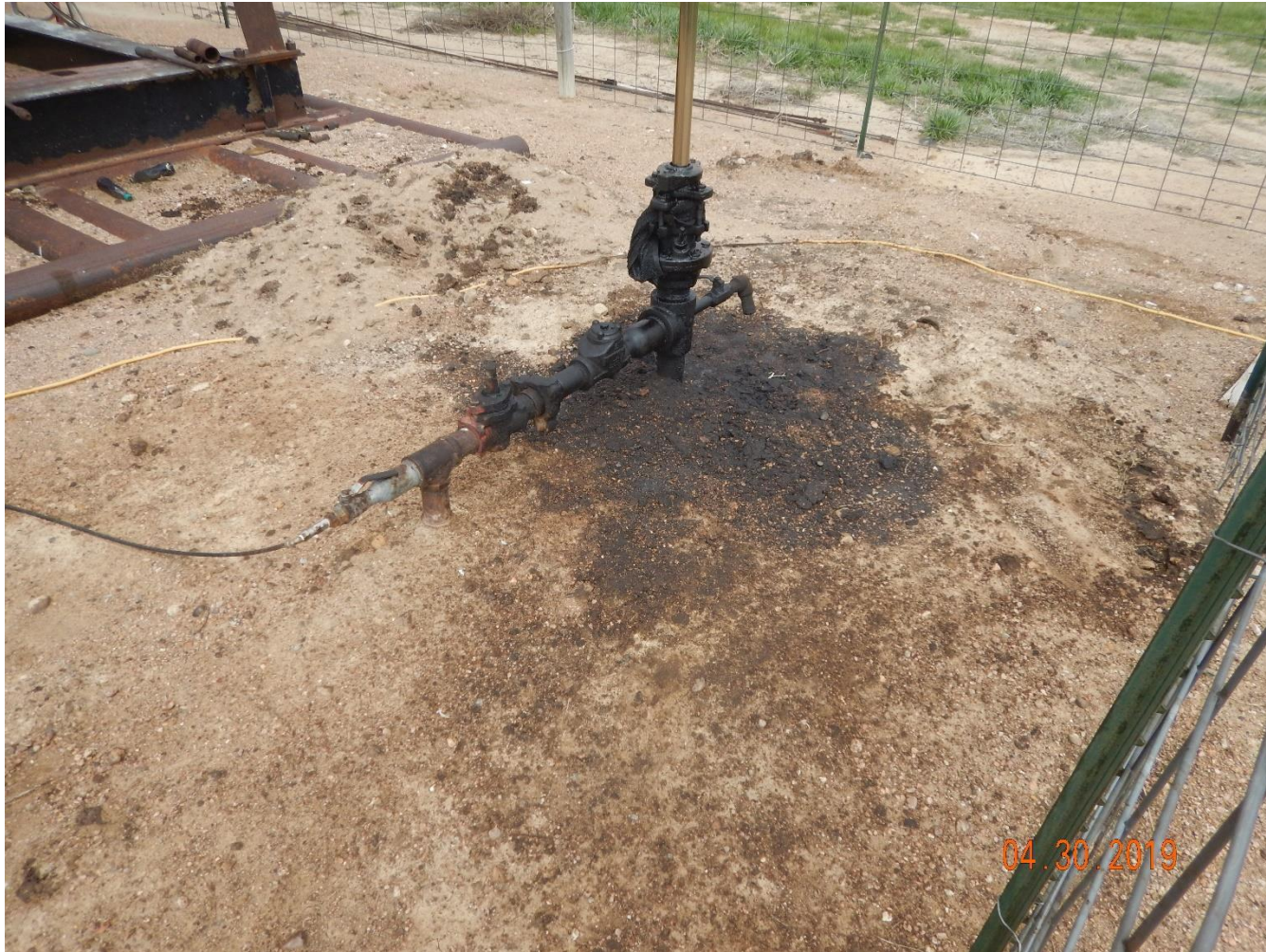
Photo 1: Photo taken from the well head. Photo shows stained/contaminated soils remain at wellhead.
