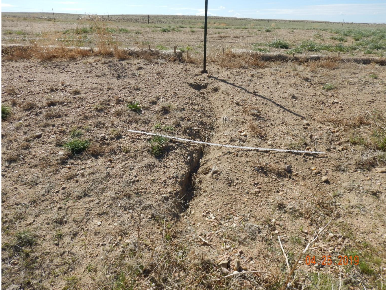
Photo 4: Photo taken from the west end of the location. Previous inspections documented erosion degradation on the western slope of the location and required operator to repair, install BMPs and monitor. Photo shows erosion degradation is beginning to recur on the west end of the location. Stormwater BMPs do not appear to be sufficient, or installed in a sufficient manner to mitigate stormwater erosion degradation. Note: Stormwater appears to be forming in areas where gaps within the wattle BMP exist.
