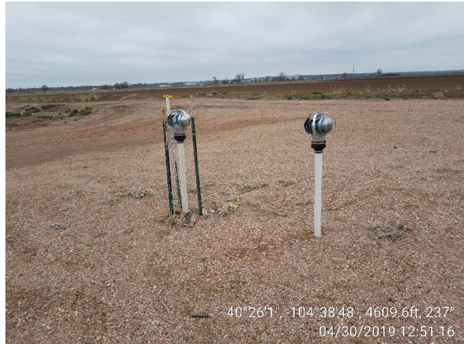
Photo 2 – Passive SVE just west of tank battery.
