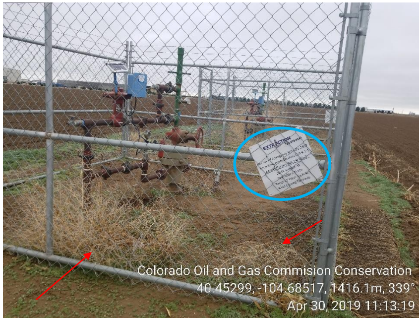
Photo 1: Wellhead; Debris needs to be removed. Wellhead sign installed.
