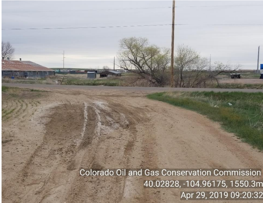
Photo 1 No tracking pad at entrance to location. Possibility of tracking sediment on to county road. Deep ruts on in road at time of inspection.
