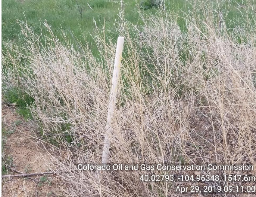
Photo 1 improperly marked Guy line anchor.
