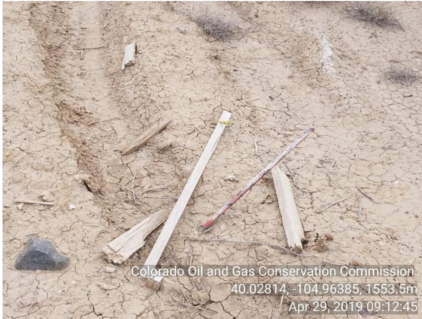
Photo 3 improperly marked Guy line anchor.
