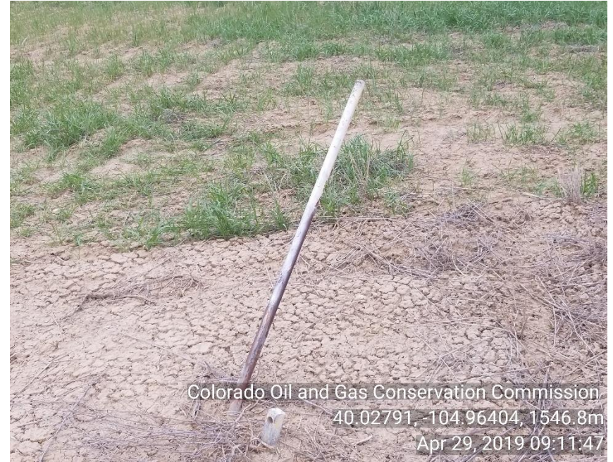
Photo 2 improperly marked Guy line anchor.
