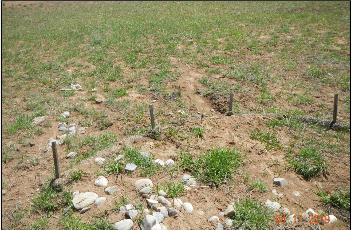
Photo 3. View of wattle at the bottom of the slope that is full of sediment.
