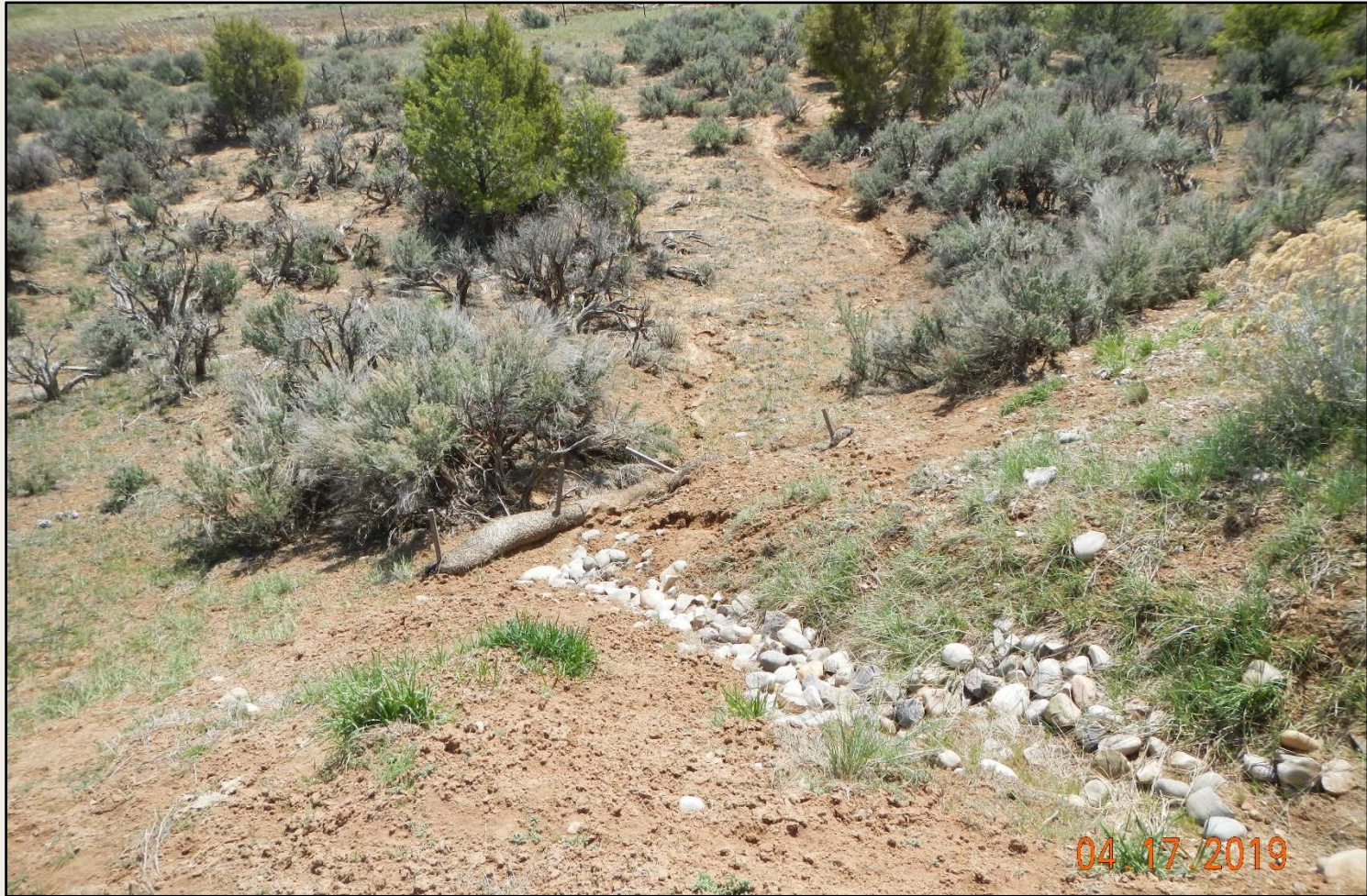
Photo 4. View of cobble within erosional channel and straw wattle that does not appear to be functioning properly.
