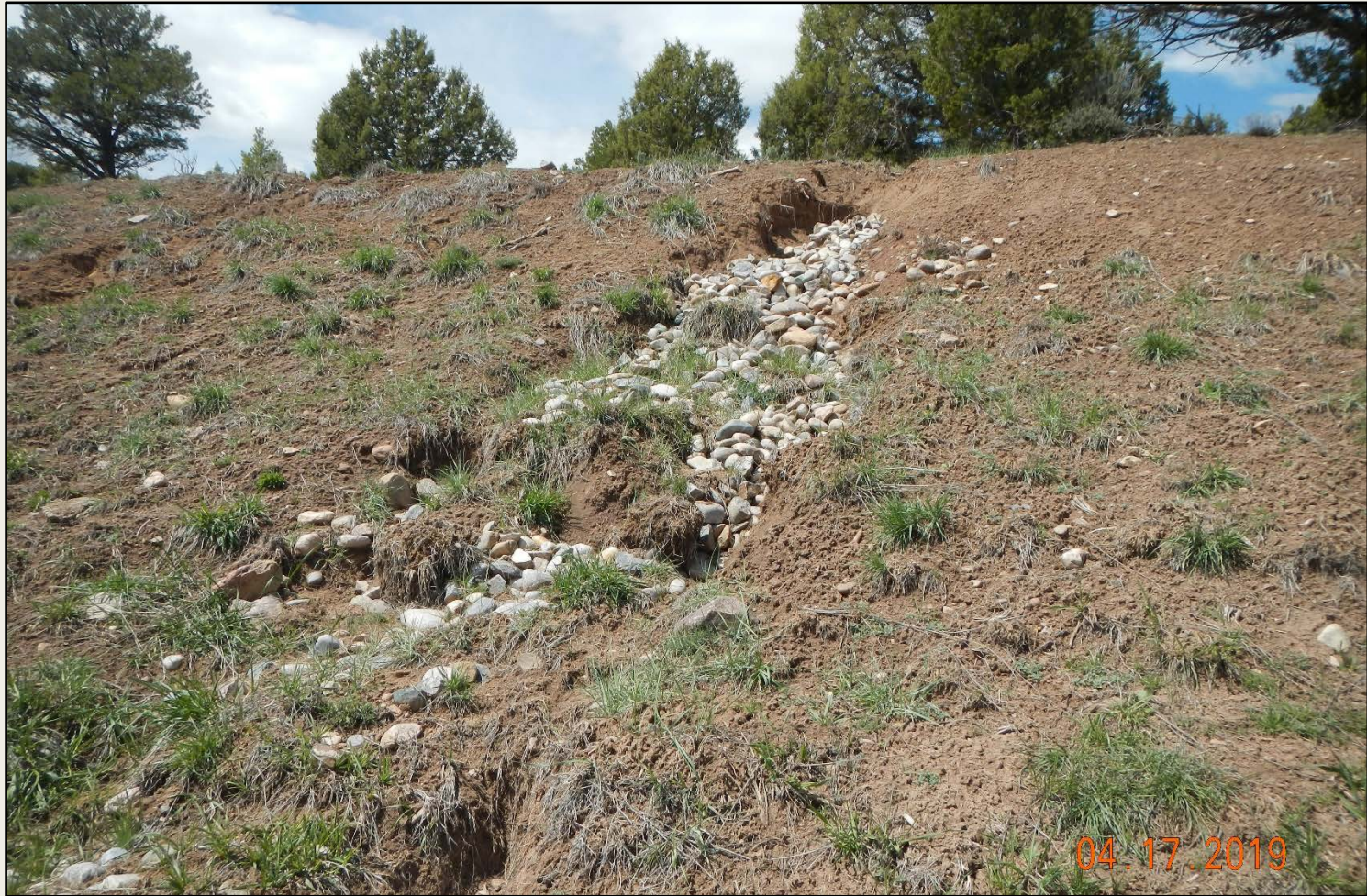
Photo 2. View of erosional channel within the western project area. Cobble placed within channel is not an effective stormwater control and erosion is continuing.
