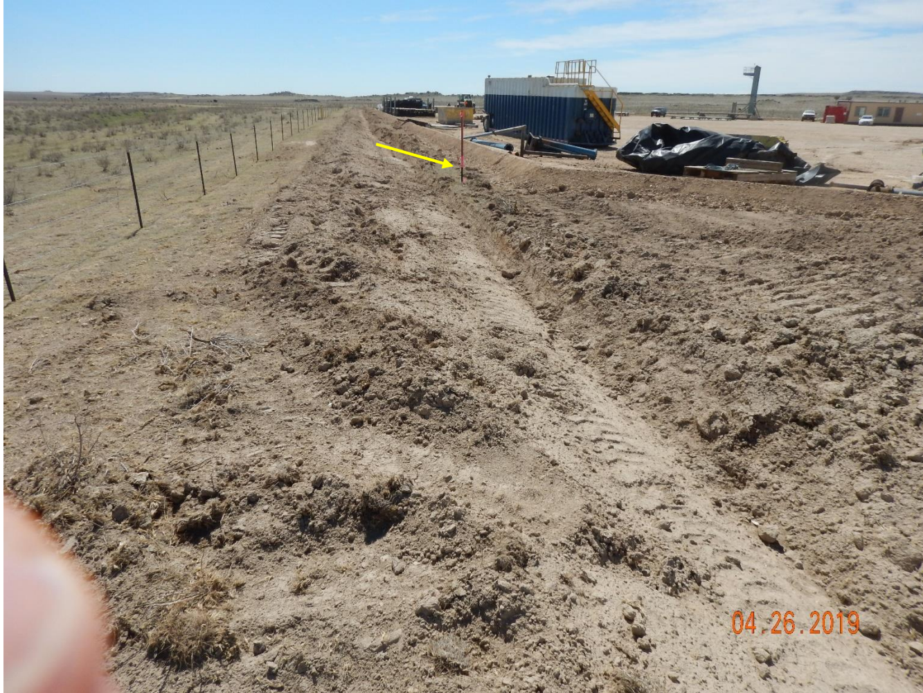
Photo 1: Photo taken from the northeast corner of the location, facing south. Photo shows survey stakes. Operator states within FIRR 401983658 that location was re-surveyed, and that the location has been constructed within the stakes. Photo shows that there area areas of the location's disturbance beyond the survey stakes on the north end of the photo.
