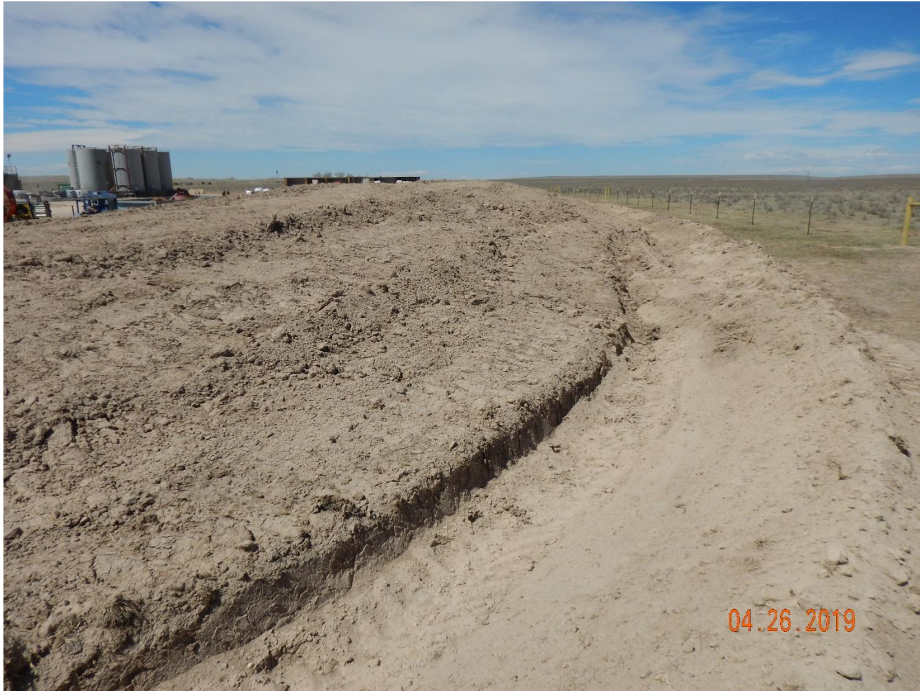
Photo 2: Photo taken from the northeast corner of the location, facing west. Operator states within FIRR 401983658 that location was re-surveyed, and that the location has been constructed within the stakes. Photo shows that there area areas of the location's disturbance beyond the survey stakes on the north end of the location.
