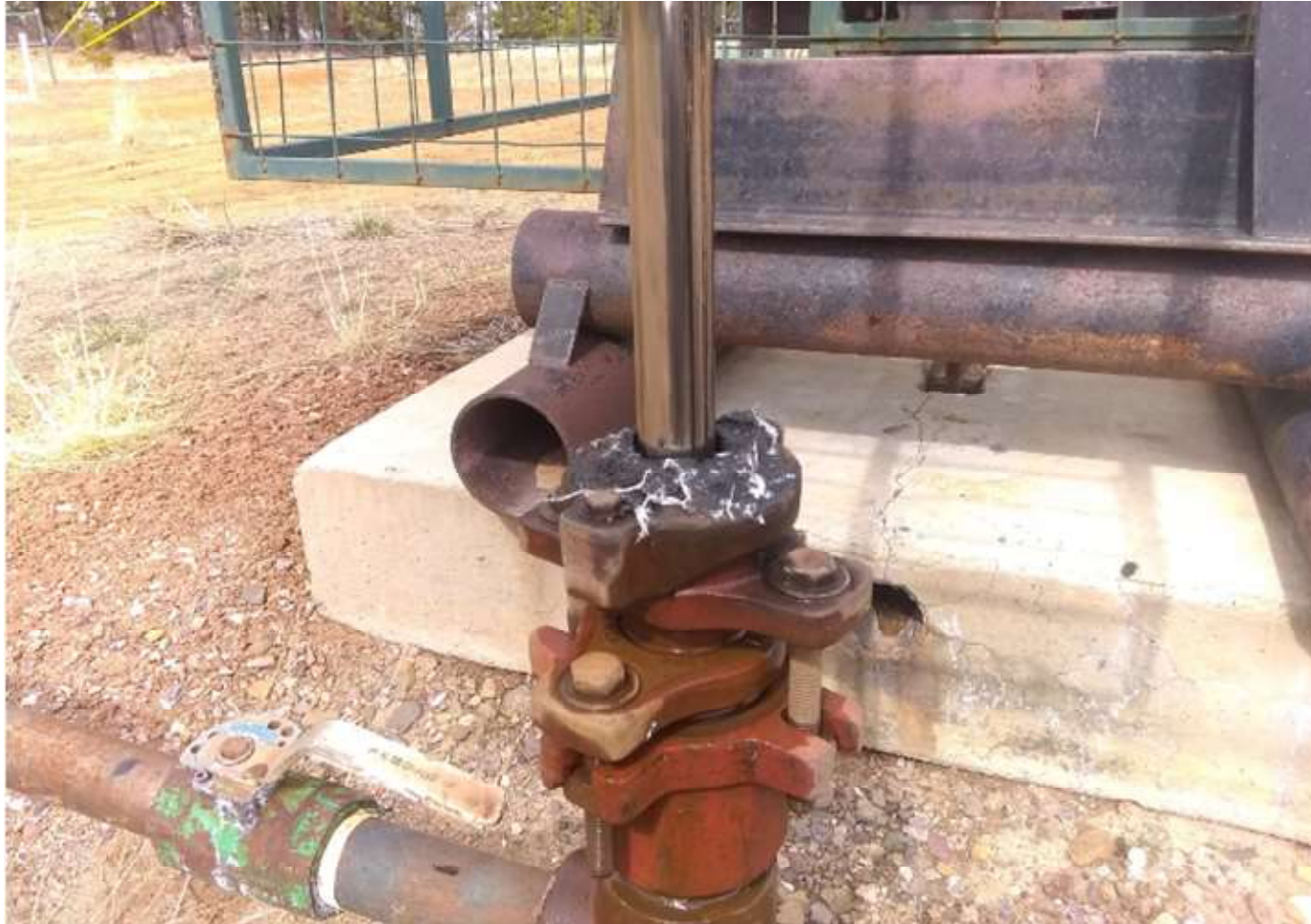
PHOTO 1: REPLACED THE PACKING TO ELIMINATE THE WATER LEAK. PACKINGS WERE SECURELY FASTENED.
