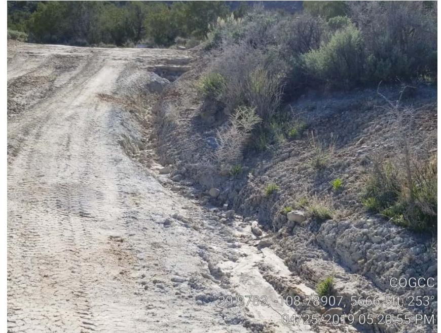
Photo 4. Storm water erosion along side of road looking away from location.
