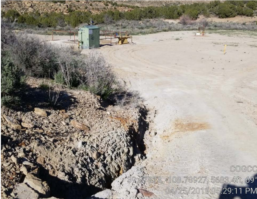
Photo 3. Storm water erosion along side of lease road entrance headed to pit.
