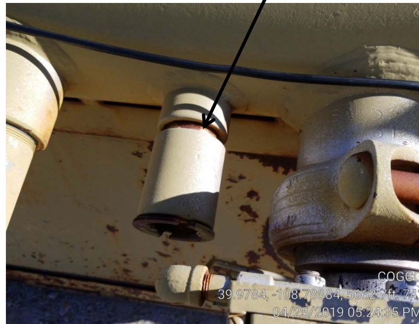
Photo 2. Separator connection leaking gas at threads.
