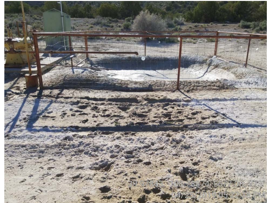
Photo 6. Storm water entered pit and spilled over berm.
