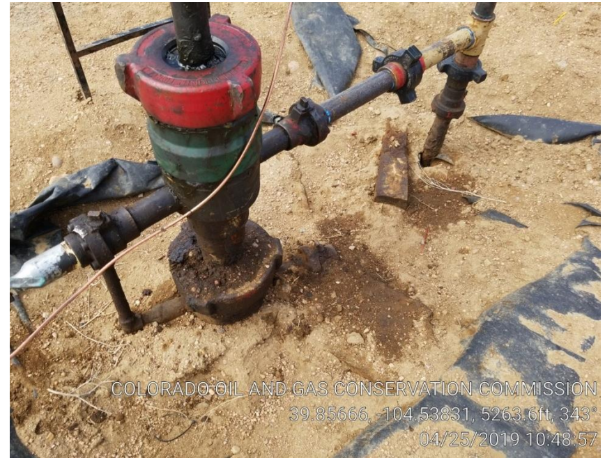
Stained soil around wellhead.
