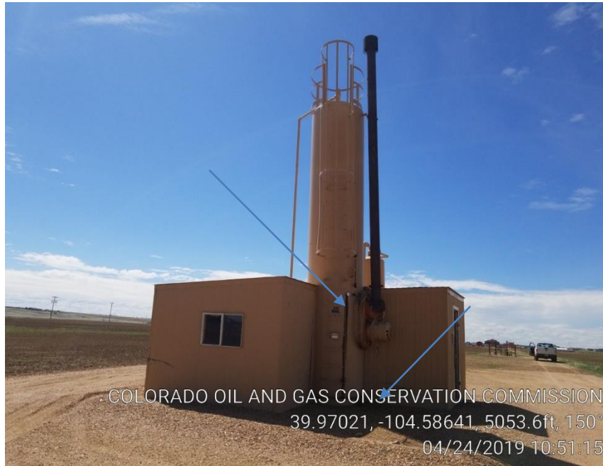
Pic 3 Possible Leak and stained soil.
