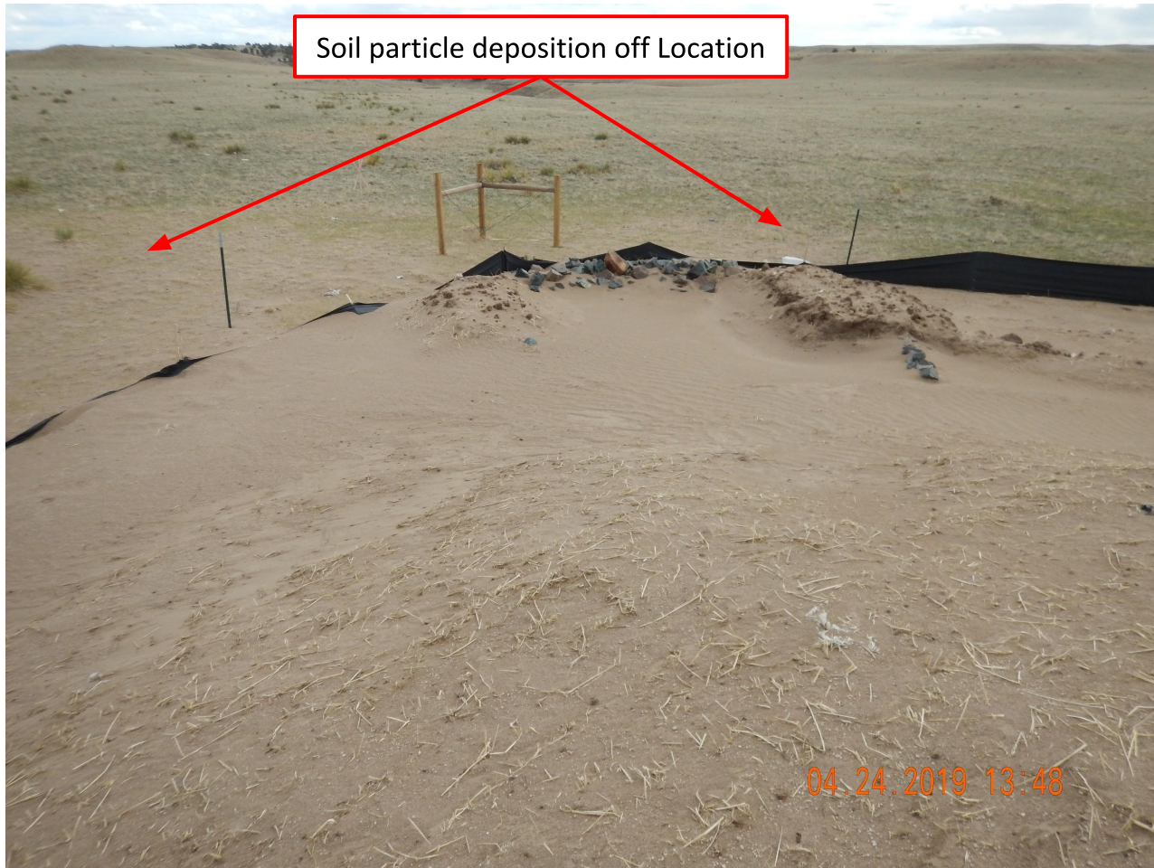
Photo 2. Photo taken from the southeastern perimeter of the location, facing South. Photo illustrates the sediment trap which has been filled in with soil particle deposition as a result of wind erosion from the well pad not being adequately stabilized. Also, it doesn't appear that the sediment trap has been adequately sized for the disturbance area.
