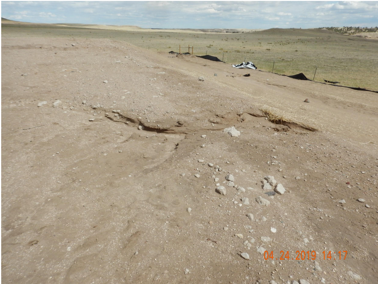
Photo 3. Photo taken from the southern location, facing East. Photo illustrates stormwater erosion which further indicates the well pad has not been adequately stabilized.
