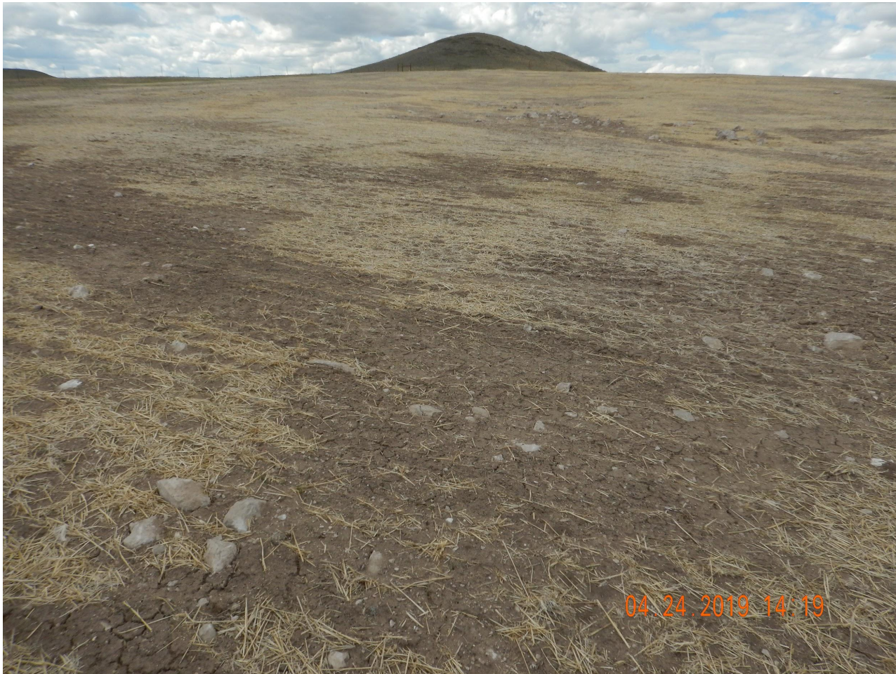
Photo 6. Photo taken from the southwestern location, facing North. This area was used for the MLVT storage during drilling operations. The area has been seeded and straw crimped with mulch. Germination was observed throughout the western area where the Operator has performed Interim Reclamation for the MLVT storage area.
