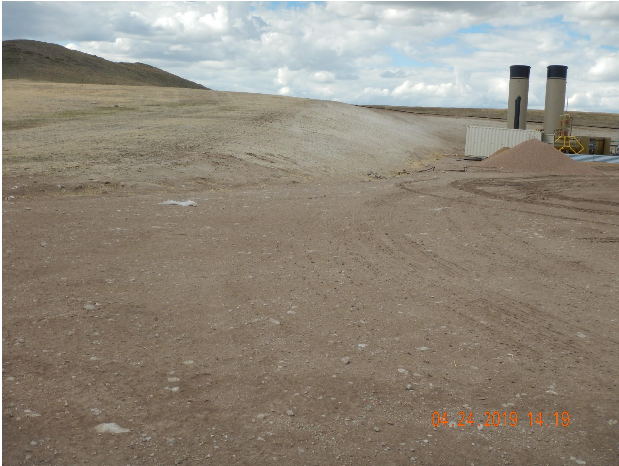
Photo 7. Photo taken from the southwestern location, facing North. Operator has the Production Facility equipment located along the northwestern well pad area. Cut slopes has been tracked with equipment, seeded and hydromulched. Wattles have been installed along the top of the northern cut slope.
