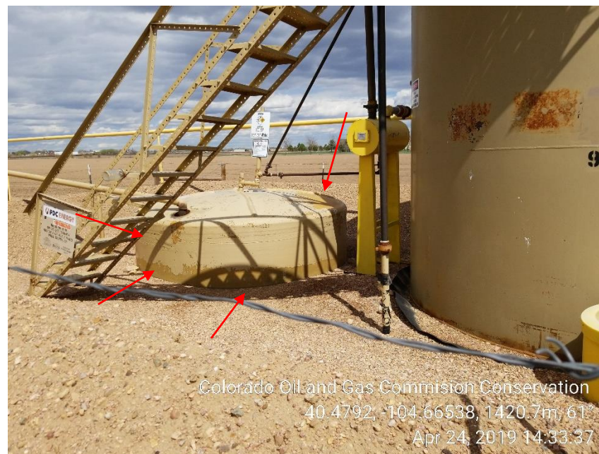
Photo 4: Chipped paint on produced water tank.
