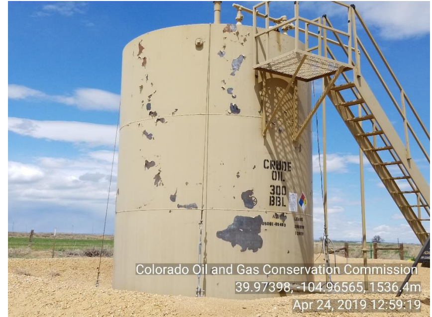
Photo 4 Tank located in view of county roads paint in disrepair.
