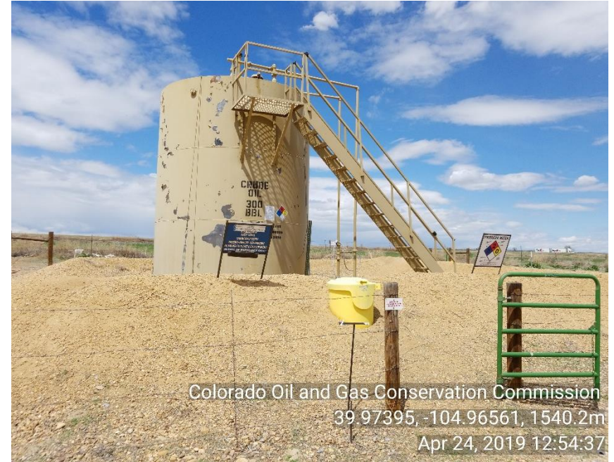
Photo 2 TNK BTYR Located in flood plain inadequate berms
