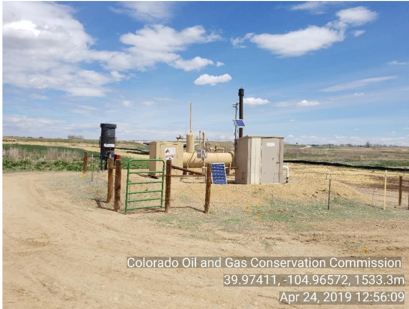
Photo 3 Sep/meter house and ECD. Located in a flood plain inadequate berms.
