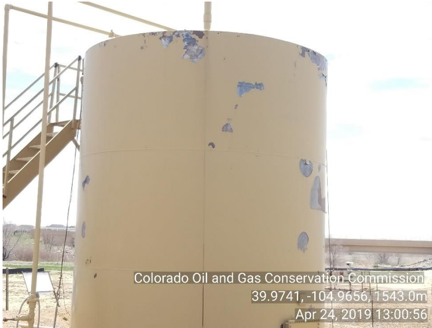
Photo 5 Tank located in view of county roads paint in disrepair.
