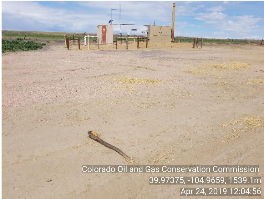
Photo 3 Unmarked Guy line anchor
