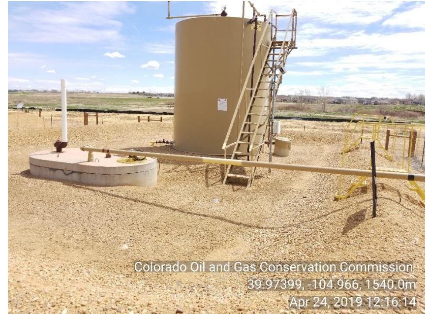
Photo 8 tanks located in flood plain not properly anchored.
