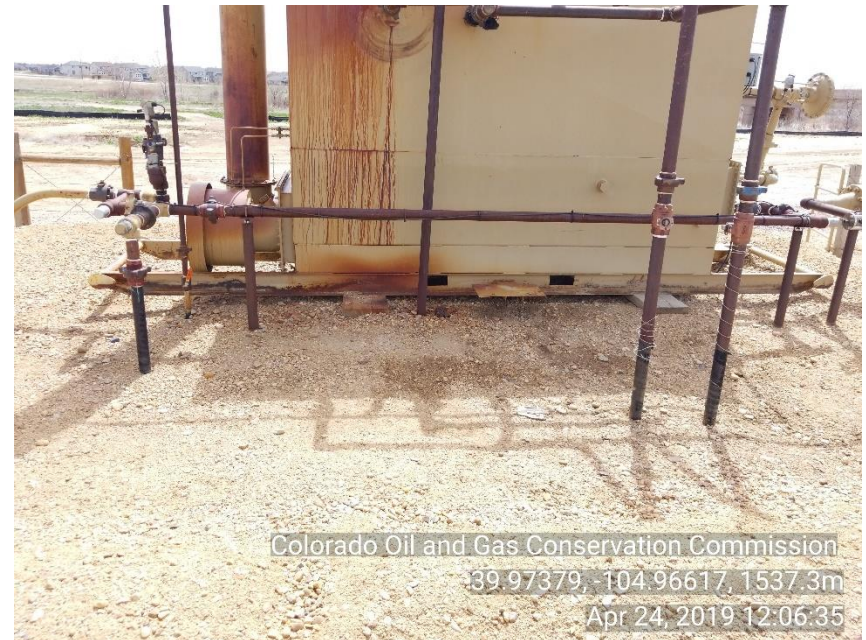
Photo 6 separator located in flood plain not properly anchored.
