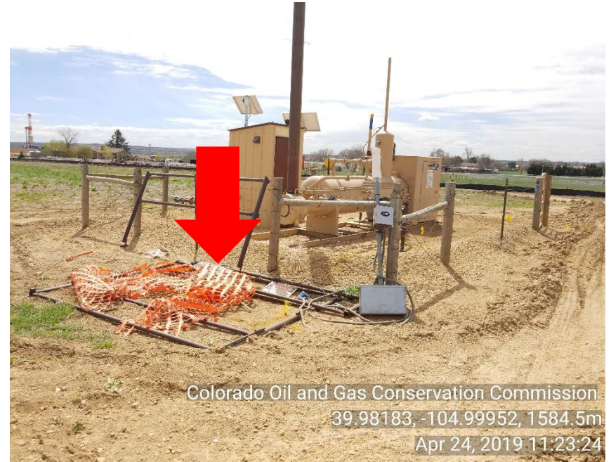
Photo 2 Sep/Meter house. Unused equipment: snow fence, telemetry equipment and steel fence.
