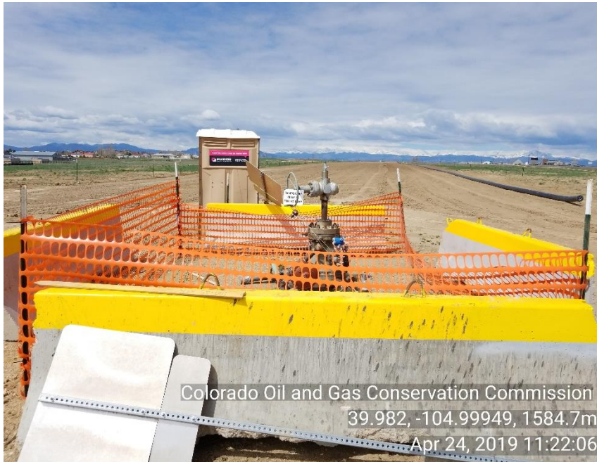
Photo 1 WH. Well is TA production equipment and flow lines have been removed from WH. Missing WH sign.
