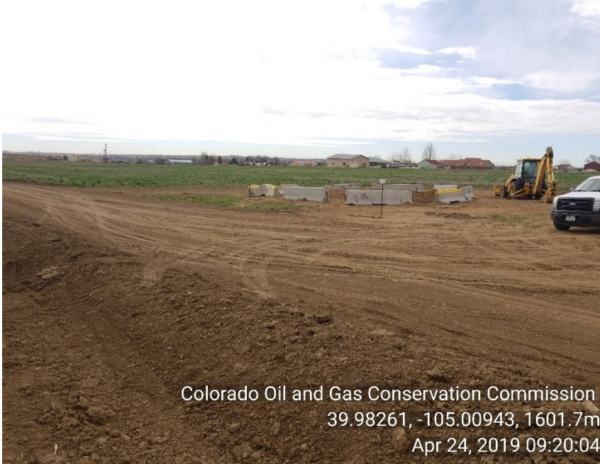
Photo 1 Well is P&A Well head appears to be removed. Storm water: No BMP's appear to be in place during the removal of production equipment during P&A process.
