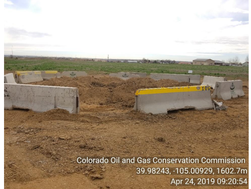
Photo 2 loc pic open hole. No BMP's appear to be in place during the removal of production equipment during P&A process.
