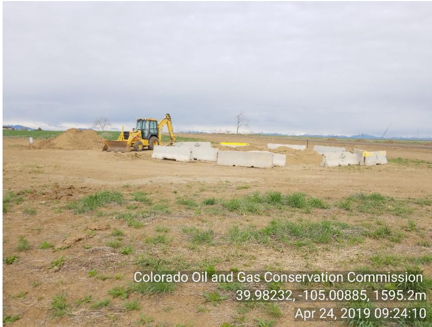
Photo 3 Loc pic. Storm water: No BMP's appear to be in place during the removal of production equipment during P&A process.
