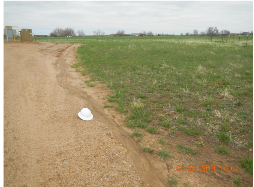
Photo 2. Photo taken from access road looking into the location, facing Northwest. Operator does not appear to have implemented and maintained Best Management Practices (BMPs) to control stormwater runoff in a manner that minimizes erosion, transport of sediment offsite, and site degradation per Rule 1002.f.(2). Operator does not appear to have implemented BMPs in accordance with good engineering practices per Rule 1002.f.(2).
