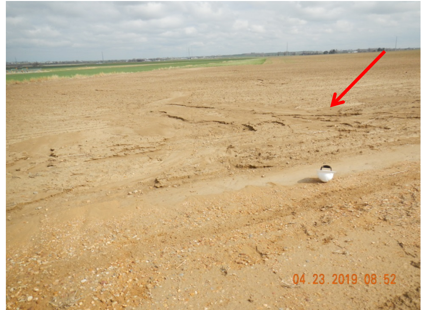
Photo 2. Photo taken from access road, facing North. Operator does not appear to have implemented and maintained Best Management Practices (BMPs) to control stormwater runoff in a manner that minimizes erosion, transport of sediment offsite, and site degradation per Rule 1002.f.(2). Operator does not appear to have implemented BMPs in accordance with good engineering practices per Rule 1002.f.(2).
