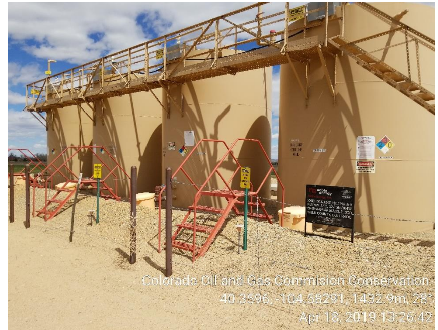
Photo 2: Centralized Tank Battery
