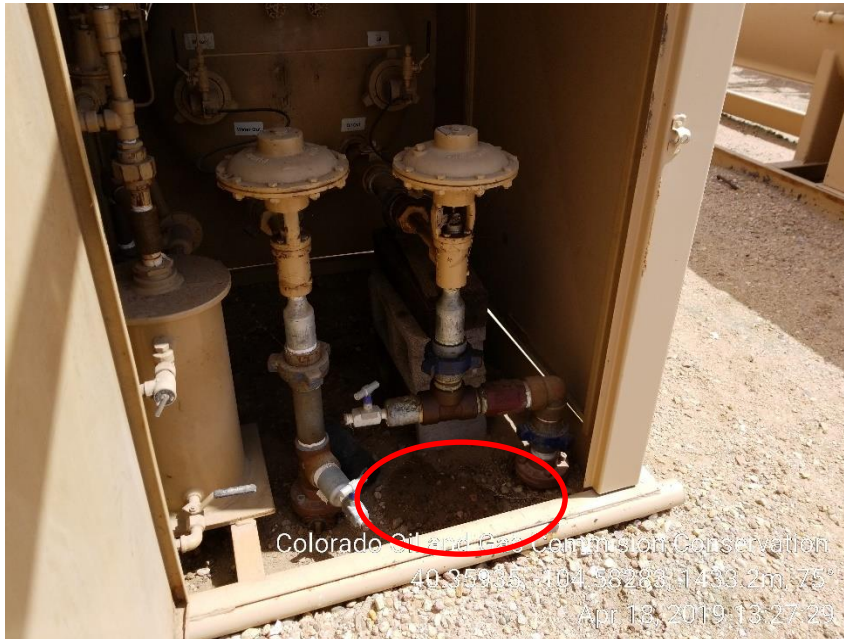
Photo 1: North separator (stained soil)
