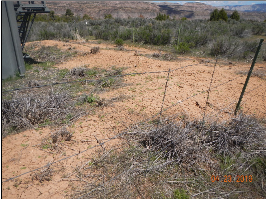
Tank berm in need of maintenance, debris in containment. .
