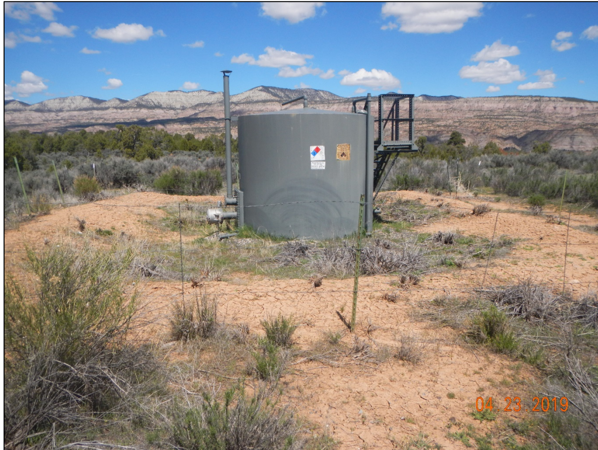
Photo of tank battery. Berm needs maintenance, Debris in Containment, labels need all current operator information
