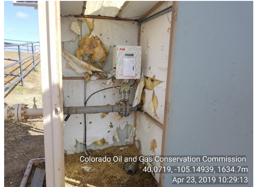
Photo 4 Meter house insulation is falling down
