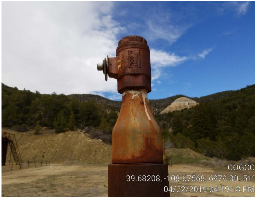
Photo 3. Gas leaking through valve.
