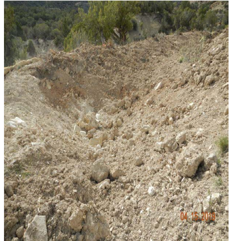
Photo#7: Sediment traps have been have been roughed in.
