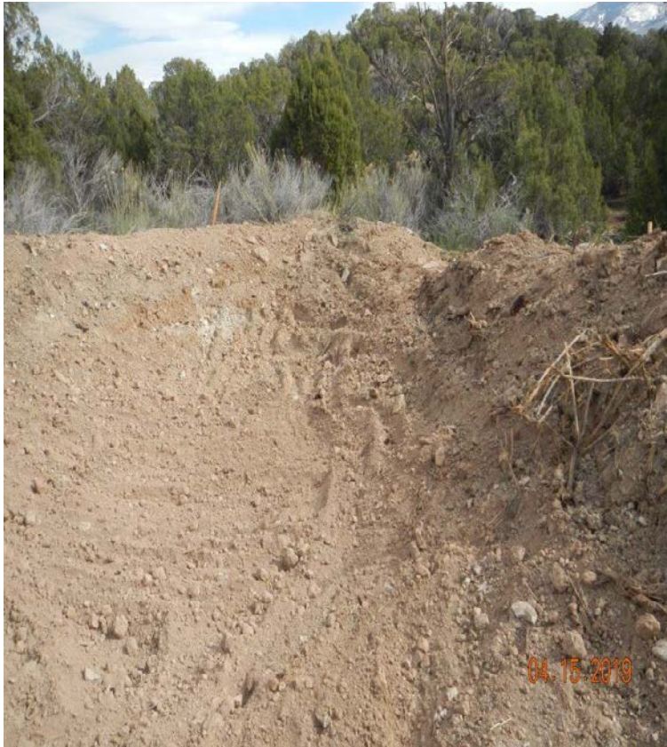
Photo#6: Sediment traps have been have been roughed in.
