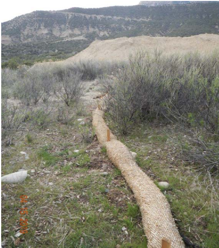
Photo#4: Wattles have been installed as perimeter Controls.
