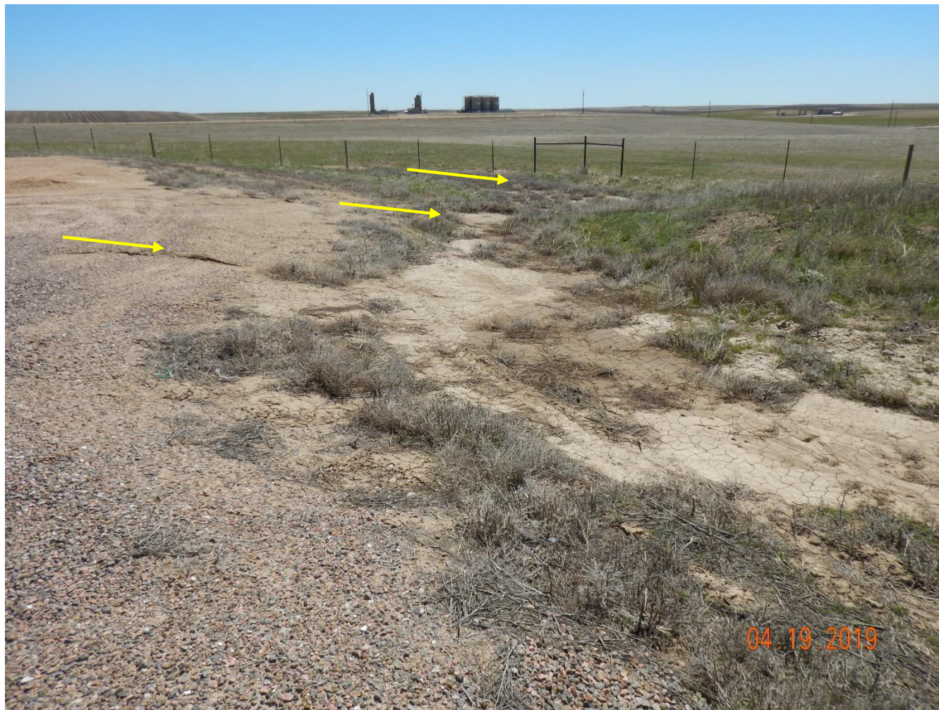
Photo 5 Photo taken from the south end of the location. Photo shows insufficient stormwater BMPs to allow for sediment laden free stormwater discharge from the location. Photo shows erosion degradation and stormwater runoff transporting sediment beyond location onto adjacent lands.
