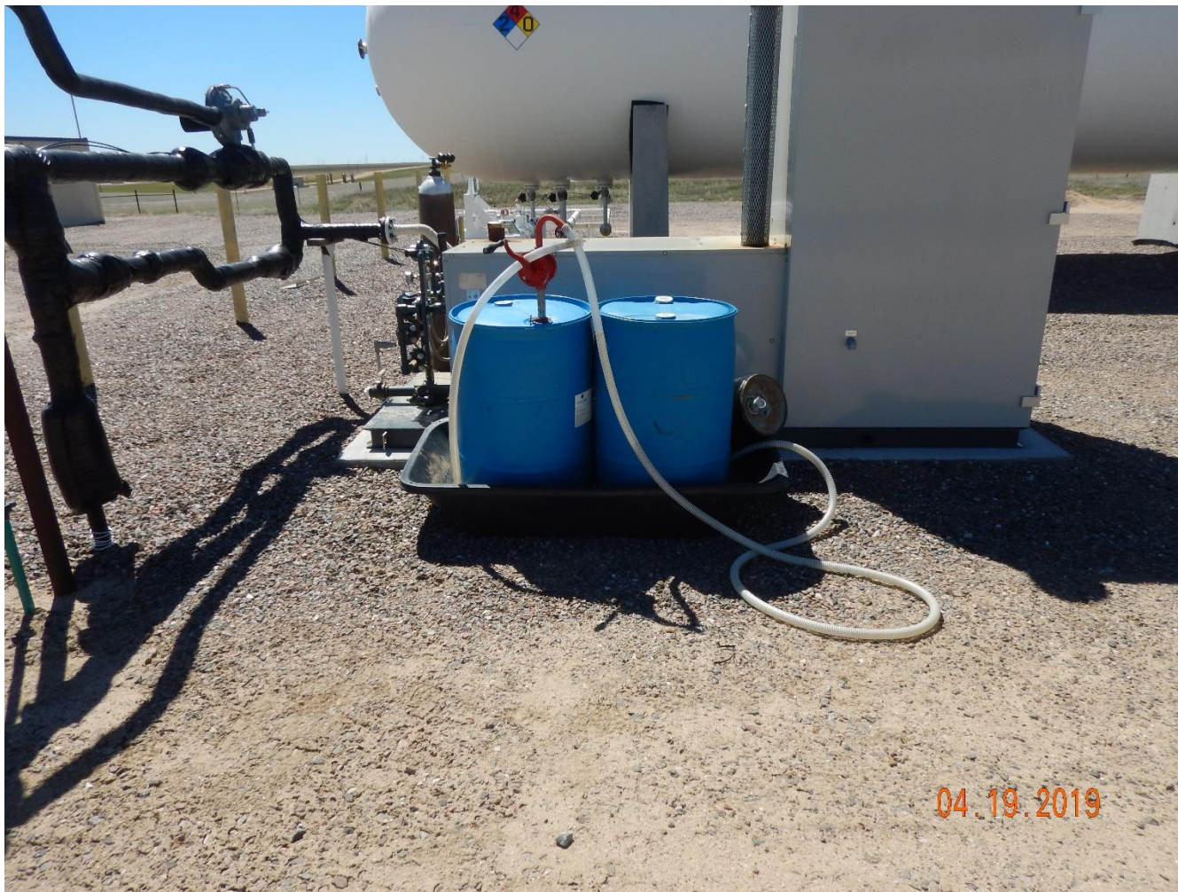
Photo 16: Photo shows barrels have been properly stored within secondary containment.
