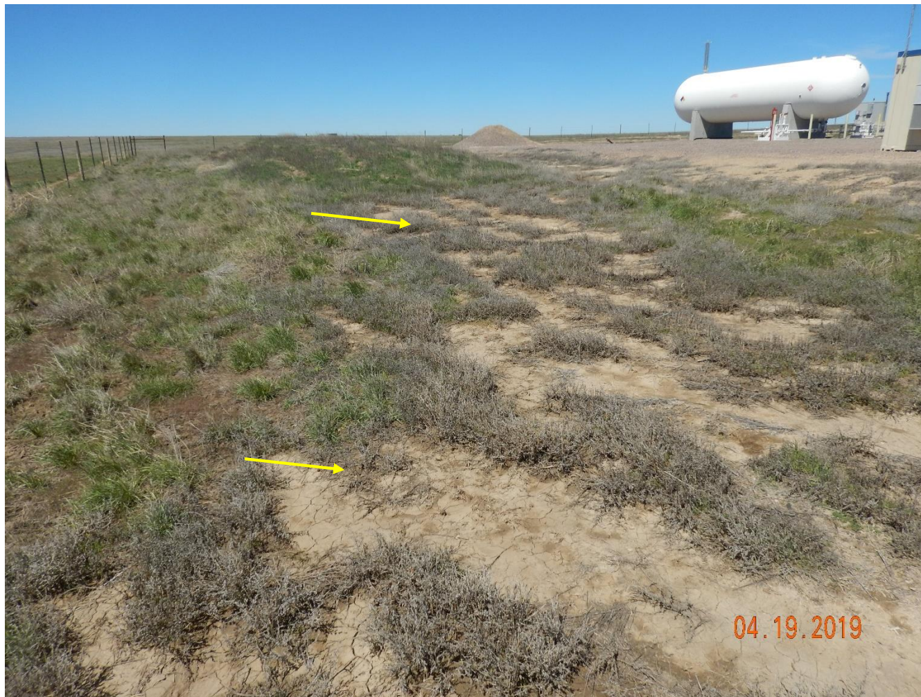
Photo 8: Photo taken from the southeast end of the location, facing west. Photo shows insufficient stormwater BMPs at the ditch to allow for sediment laden free stormwater discharge from the location. Photo also shows sediment deposition on the interim area.
