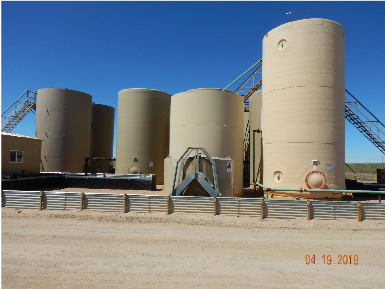
Photo 18: Photo taken from the location, facing west. Photo shows the ten (10) tanks at the battery. Tanks appears have tank contents and NFPA labelling, however, tanks appear to be missing capacity labeling in accordance with 210.d
