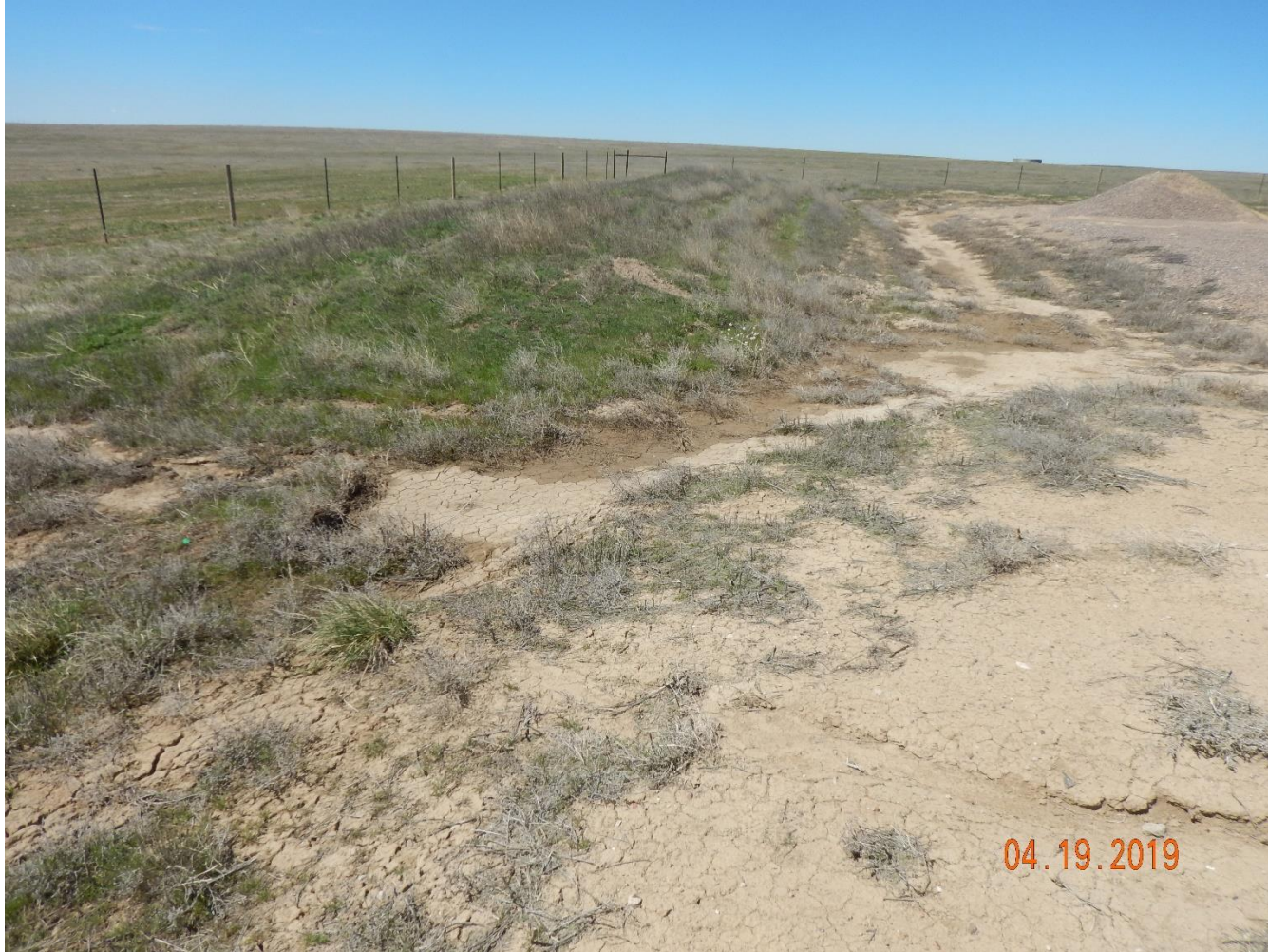
Photo 6: Photo taken from the south end of the location. Photo shows insufficient stormwater BMPs at the ditch to allow for sediment laden free stormwater discharge from the location.
