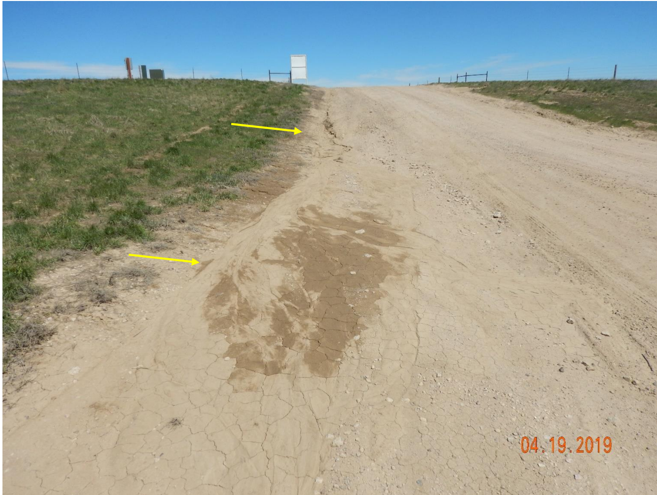
Photo 20: Photo taken from the location, facing north. Photo shows erosion degradation on access road.
