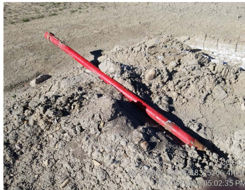
Photo 2. Deadman marker bent over.
