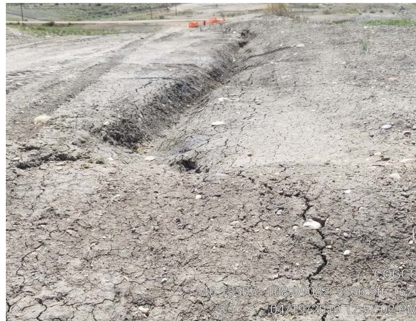
Photo 2. Breached stormwater edge berm on south edge of location.
