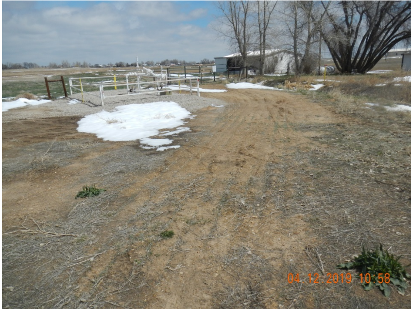
Photo 1. Photo taken from the access road off CR 8, facing Northeast. Appears Operator has performed final reclamation activities at the access road and facility with the evidence of drill rows, straw crimped mulch and some revegetation. However, parts of the reclamation is not at percent cover and has non-uniform establishment of vegetation cover.
