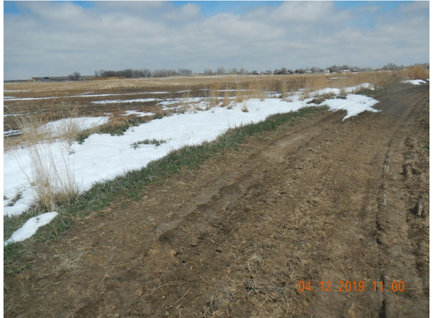
Photo 2. Photo taken from the existing land owner access road looking towards the location, facing North. Appears Operator has performed final reclamation activities at the location and northern part of the access road with the evidence of drill rows matching the adjacent cropland.
