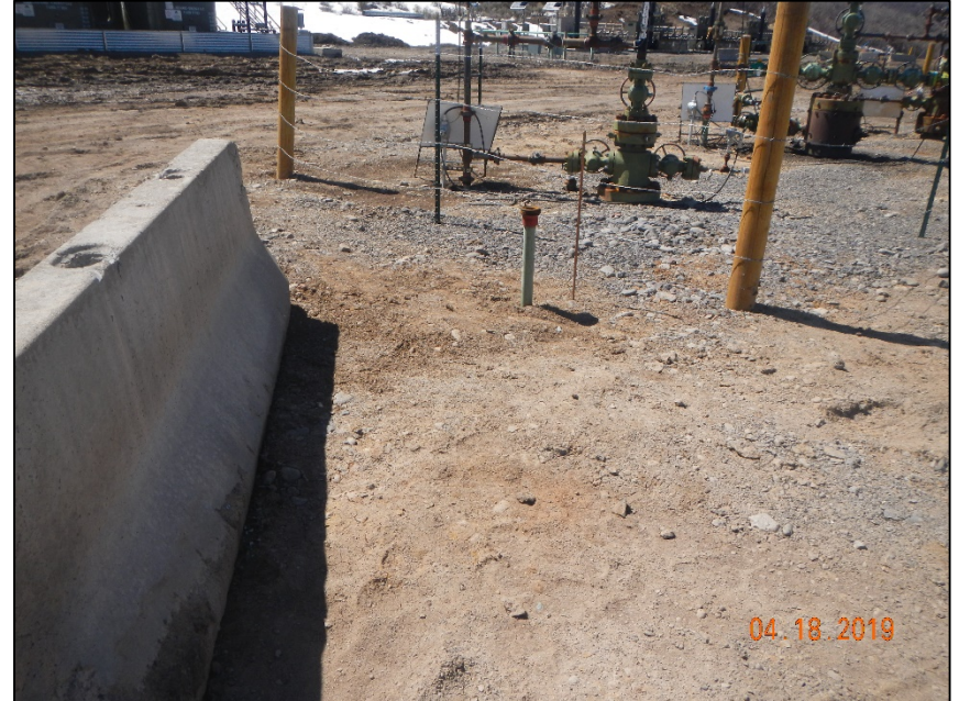
Unmarked riser by wellhead
