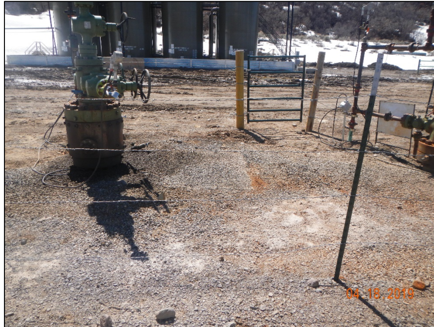
Photo of Wellheads with soil stain, Full white chemical container and containment removed.
