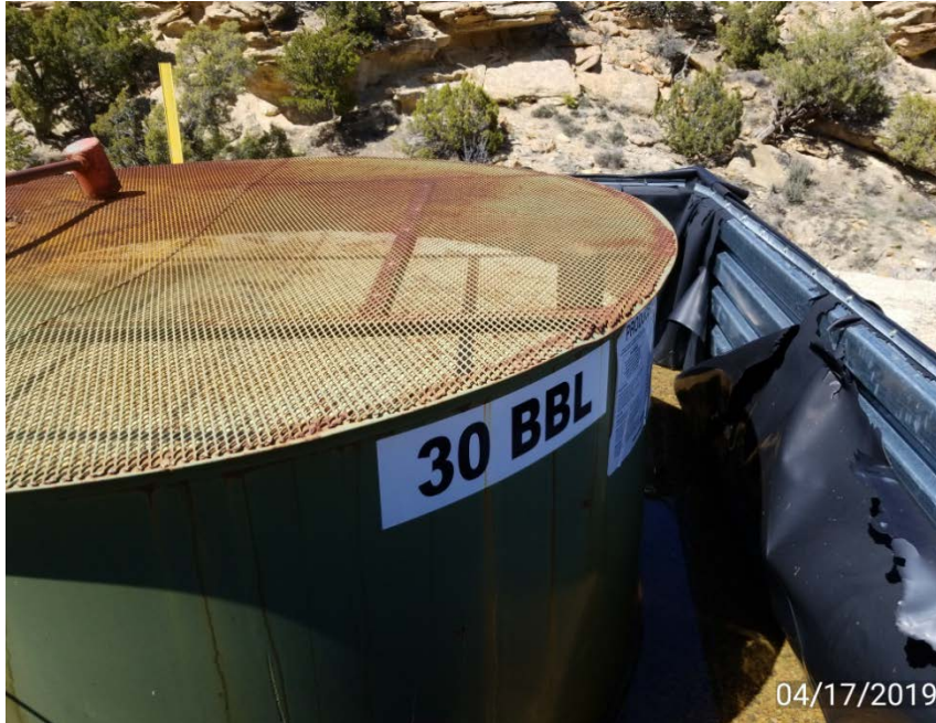
Photo 3. Torn secondary containment liner.
