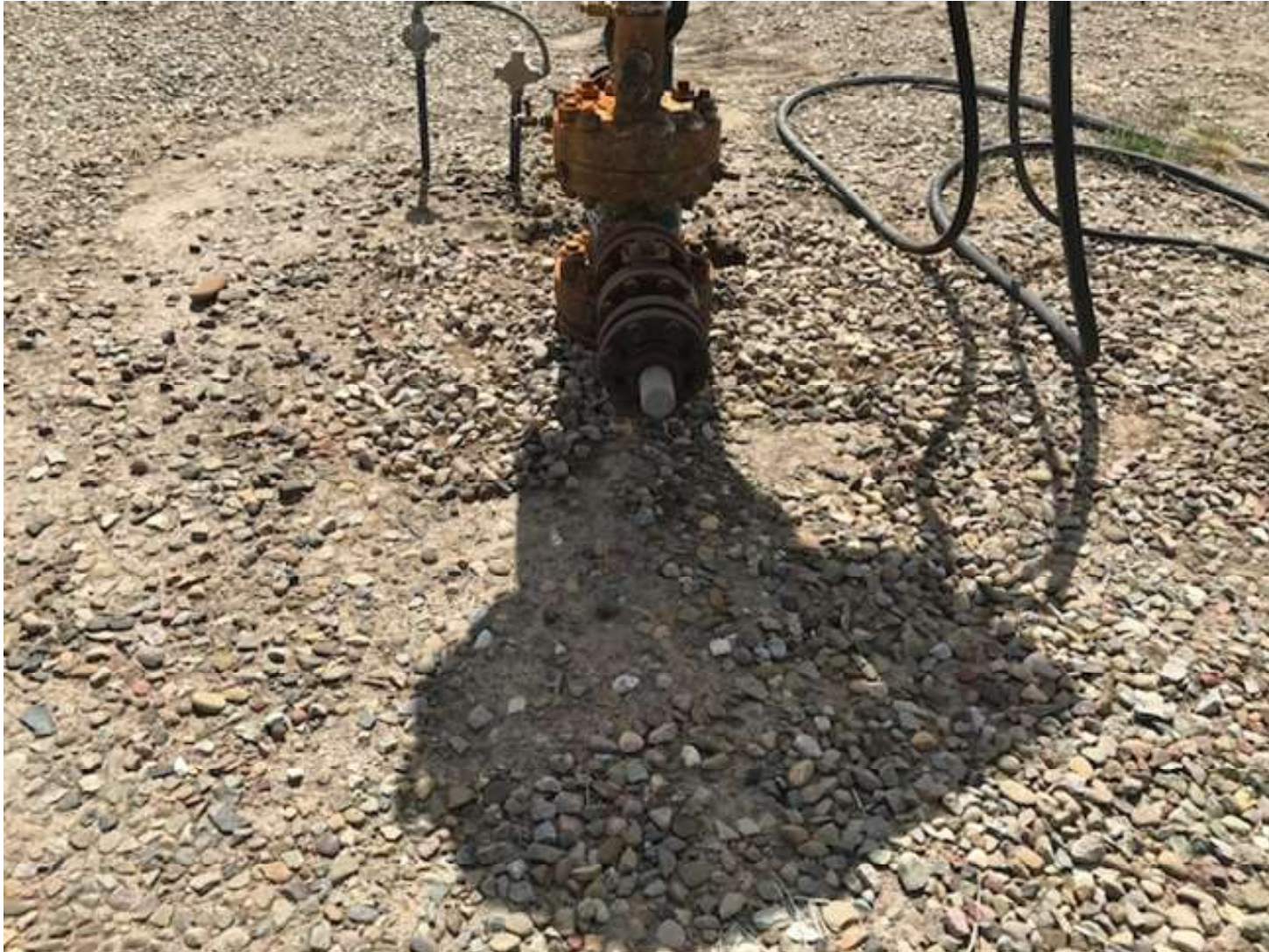
PHOTO 1: THE IMPACTED SOIL AROUND THE WELL HEAD WAS REMOVED FROM THE LOCATION. ALL VALVES AND FITTINGS WERE SECURELY FASTENED.
