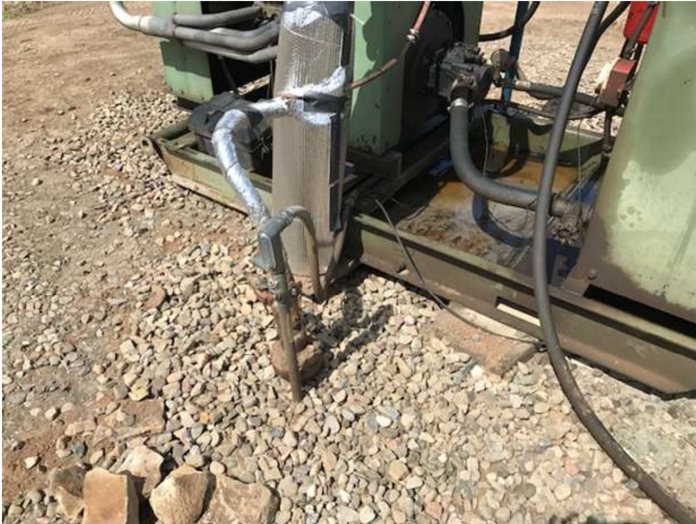
PHOTO 2: THE IMPACTED SOIL NEXT TO THE ENGINE SKID WAS REMOVED FROM THE LOCATION. THE FLUID ACCUMULATION WAS REMOVED FROM THE ENGINE SKID CONTAINMENT.
