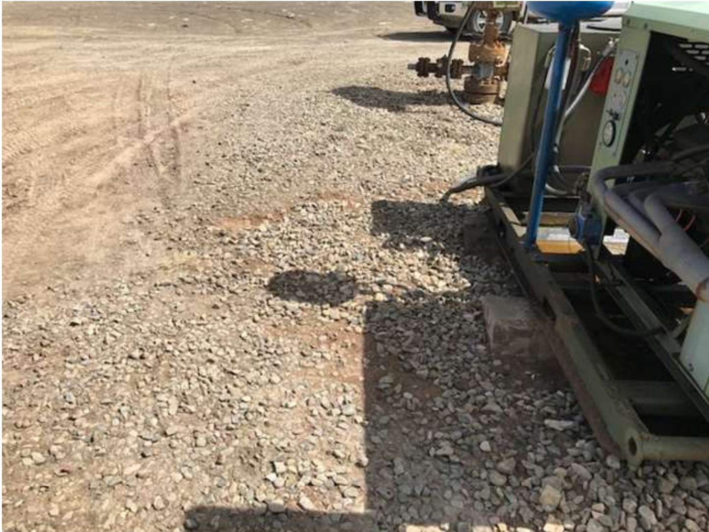
PHOTO 4: THE IMPACTED SOIL NEXT TO THE ENGINE SKID WAS REMOVED FROM THE LOCATION.
