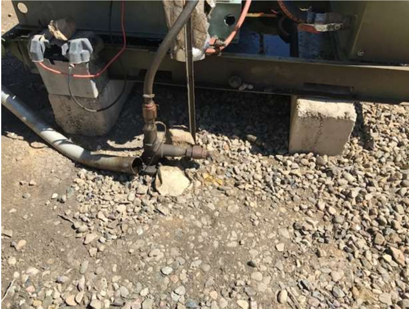
PHOTO 2: THE IMPACTED SOIL AROUND THE ENGINE SKID WAS REMOVED FROM LOCATION.
