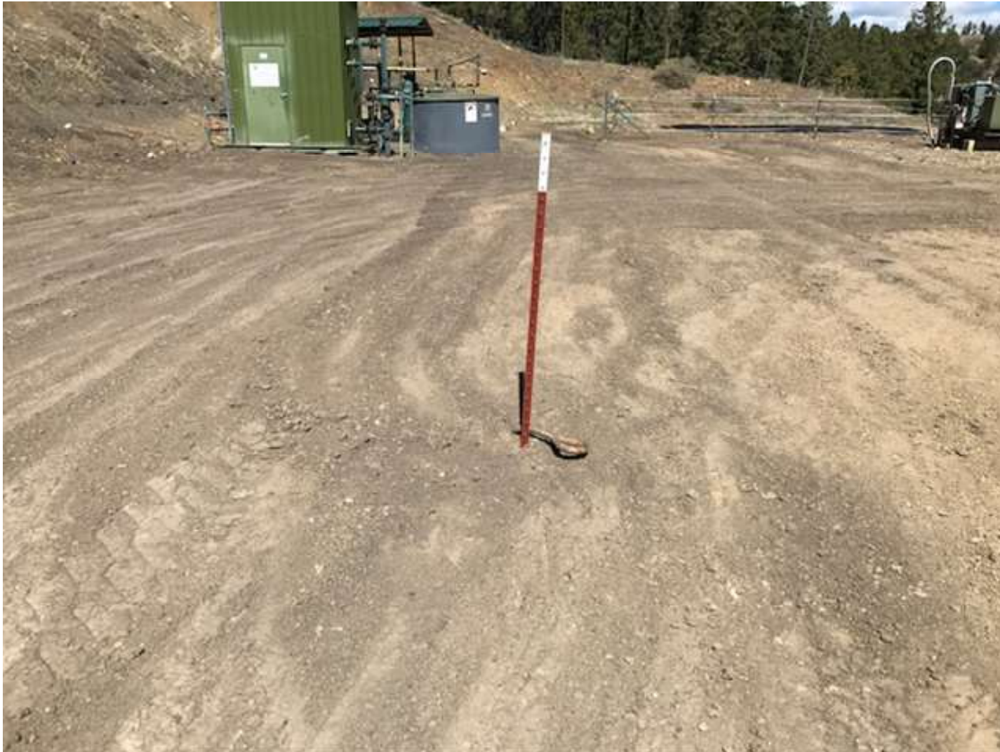
PHOTO 4: THE DEADMAN ANCHORS WERE MARKED WITH RED POSTS.
