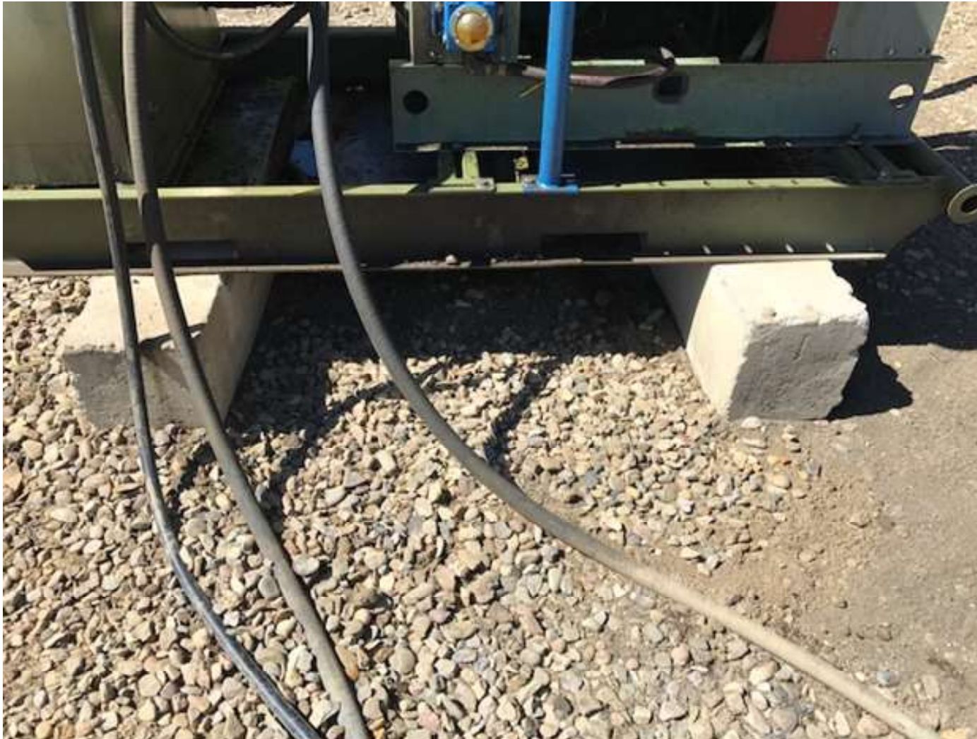
PHOTO 3: THE IMPACTED SOIL AROUND THE ENGINE SKID WAS REMOVED FROM LOCATION.
