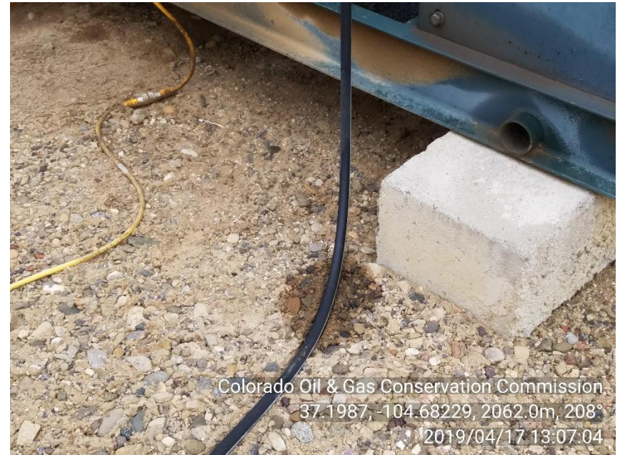
PHOTO 6: IMPACTED SOIL ON SOUTH SIDE OF COMPRESSOR PRIME MOVER SKID.
