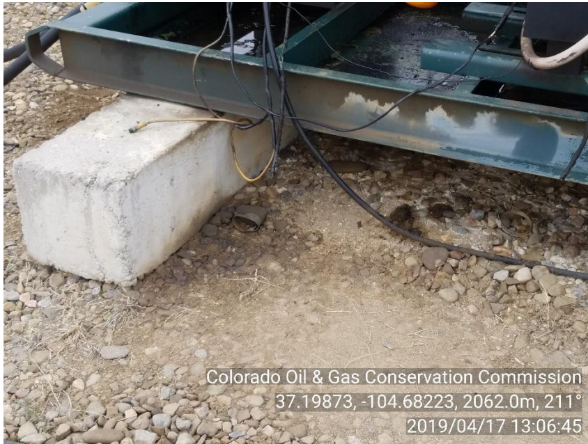
PHOTO 5: IMPACTED SOIL ON NORTH SIDE OF COMPRESSOR PRIME MOVER SKID.
