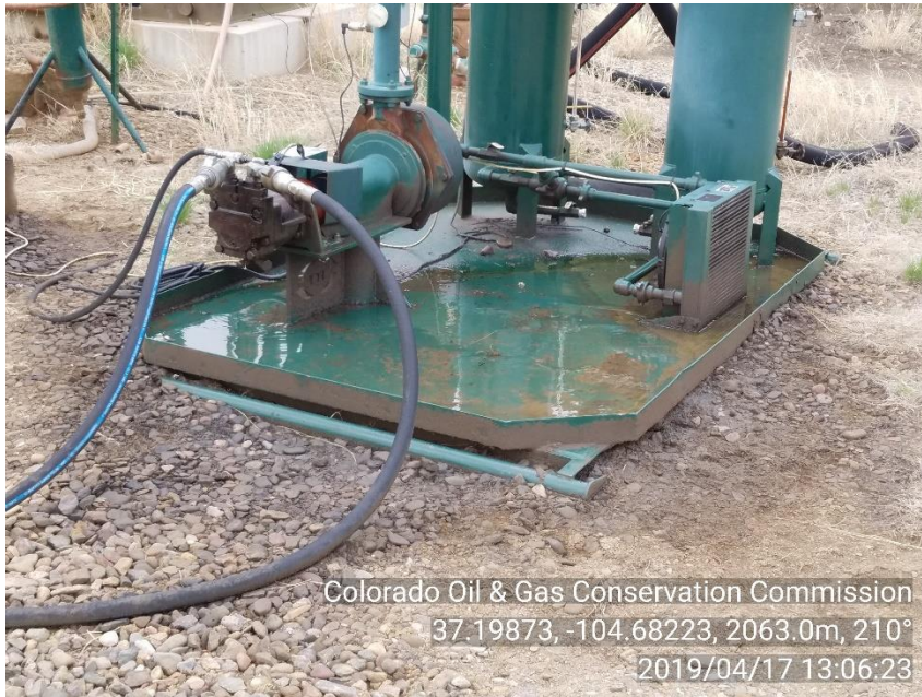
PHOTO 3: IMPACTED SOIL ALL AROUND COMPRESSOR SKID
