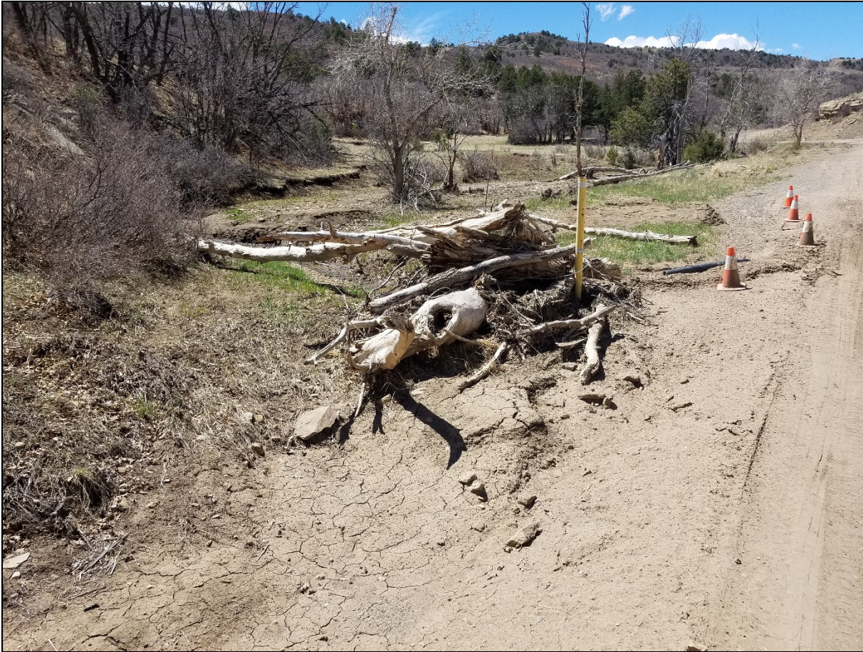
Photo 2. The culvert has been plugged up at the stream crossing causing stormwater to flow down the road.
