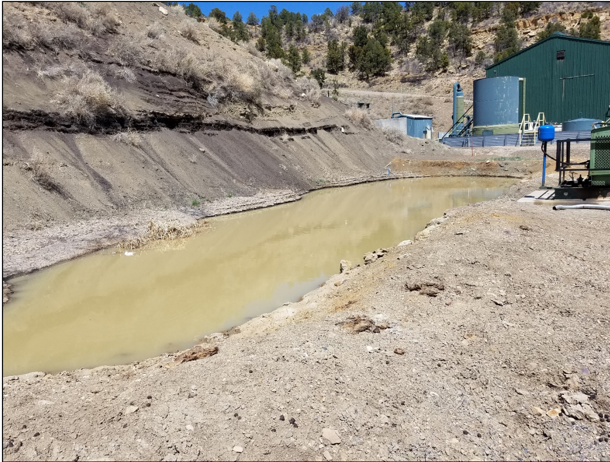
Photo 9. Pit at the location has 2ft. Freeboard and marker.
