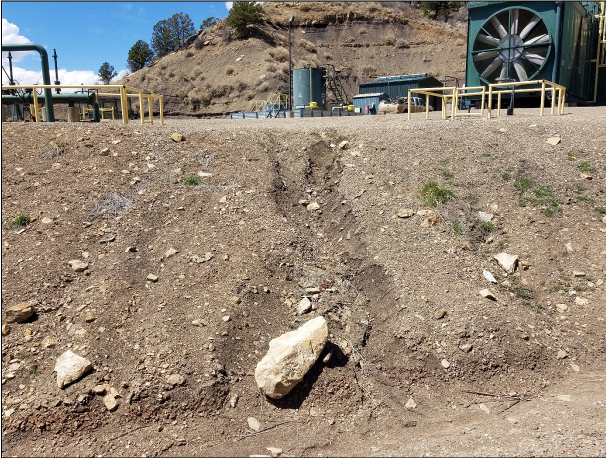
Photo 6. There are erosion issues off the east side of the pad.
