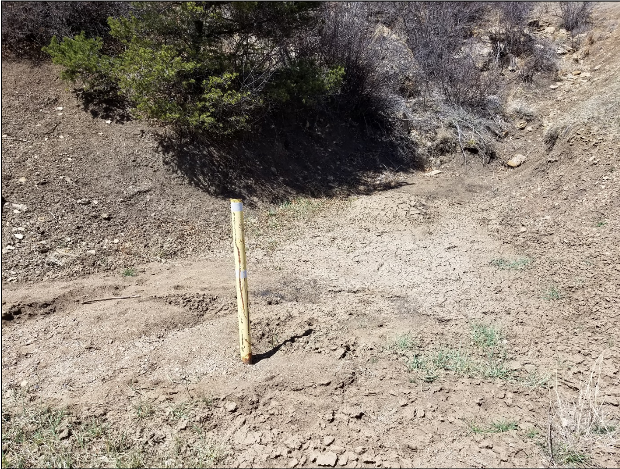
Photo 3. Another culvert up the main road is filled in with sediment.
