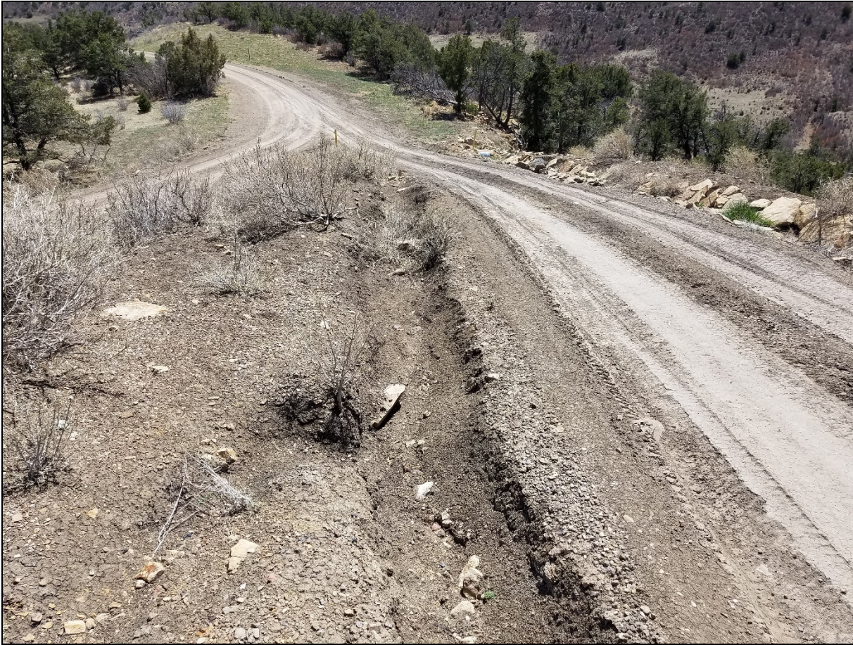
Photo 10. South access road has signs of erosion. BMP's are needed to prevent further erosion.
