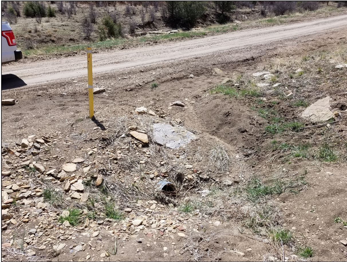
Photo 4. Further up the road is another culvert that is halfway full of sediment.
