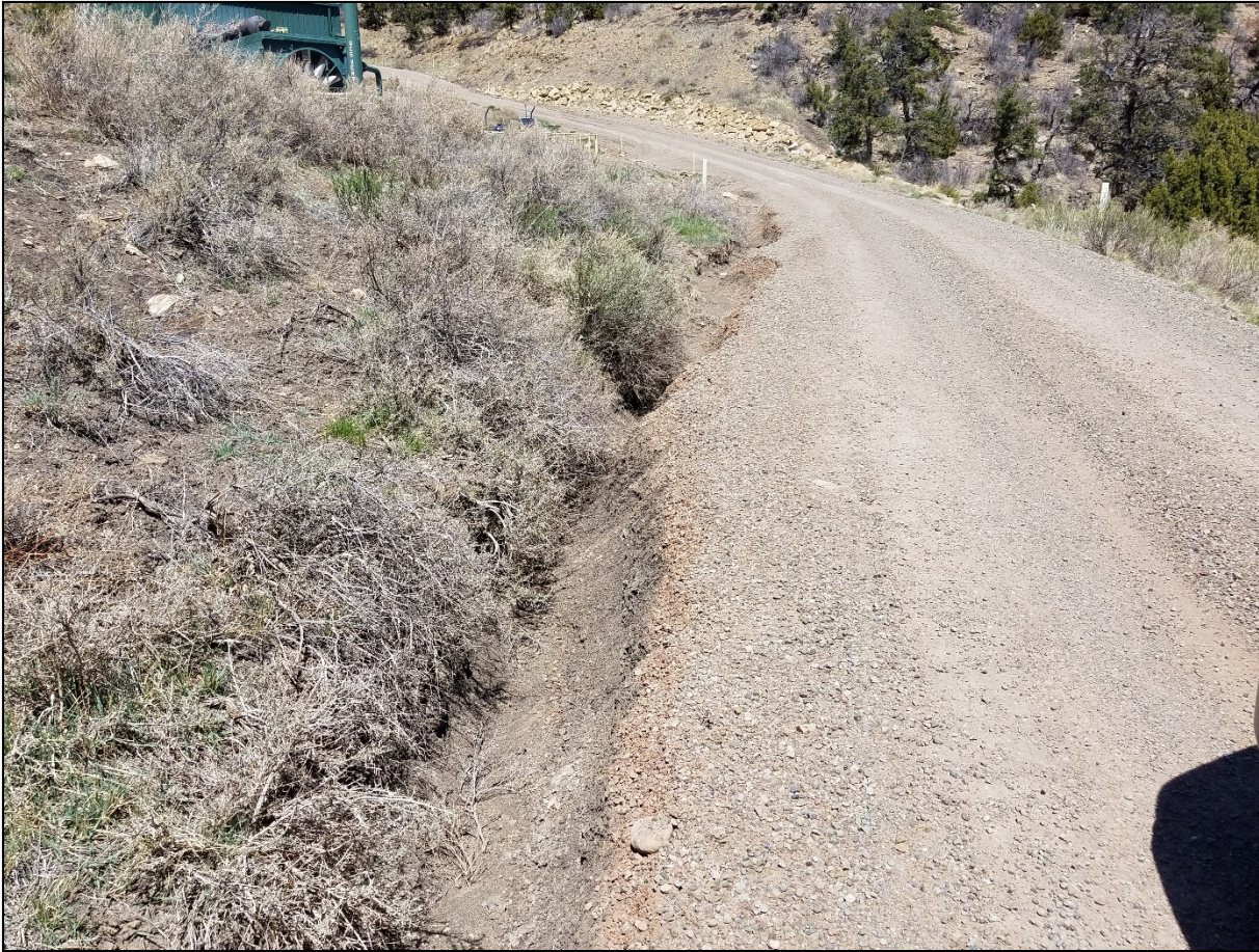
Photo 5. Erosion has deepened the side of the access road near the location. BMP's are needed to prevent further erosion.
