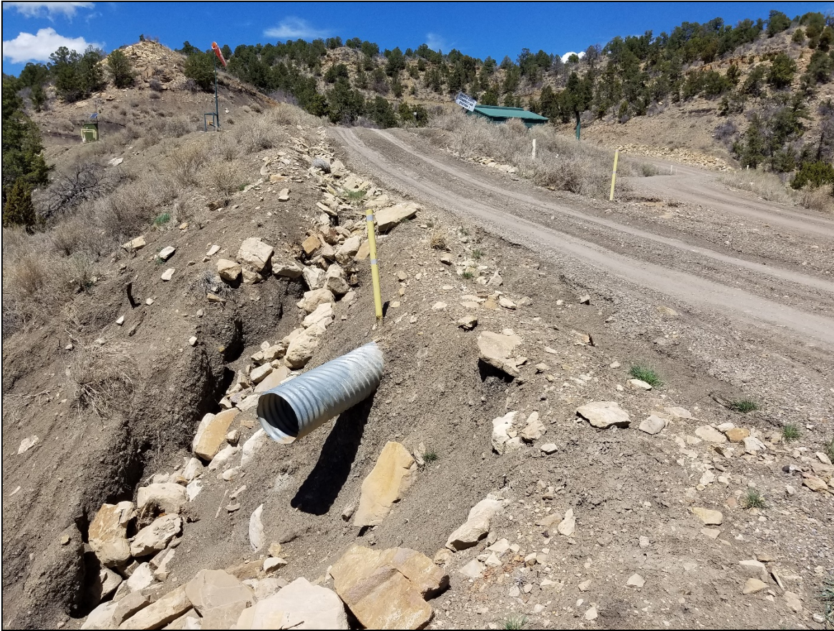
Photo 11. The culvert at the access road has had erosion issues. More rip/rap may be needed in this area.
