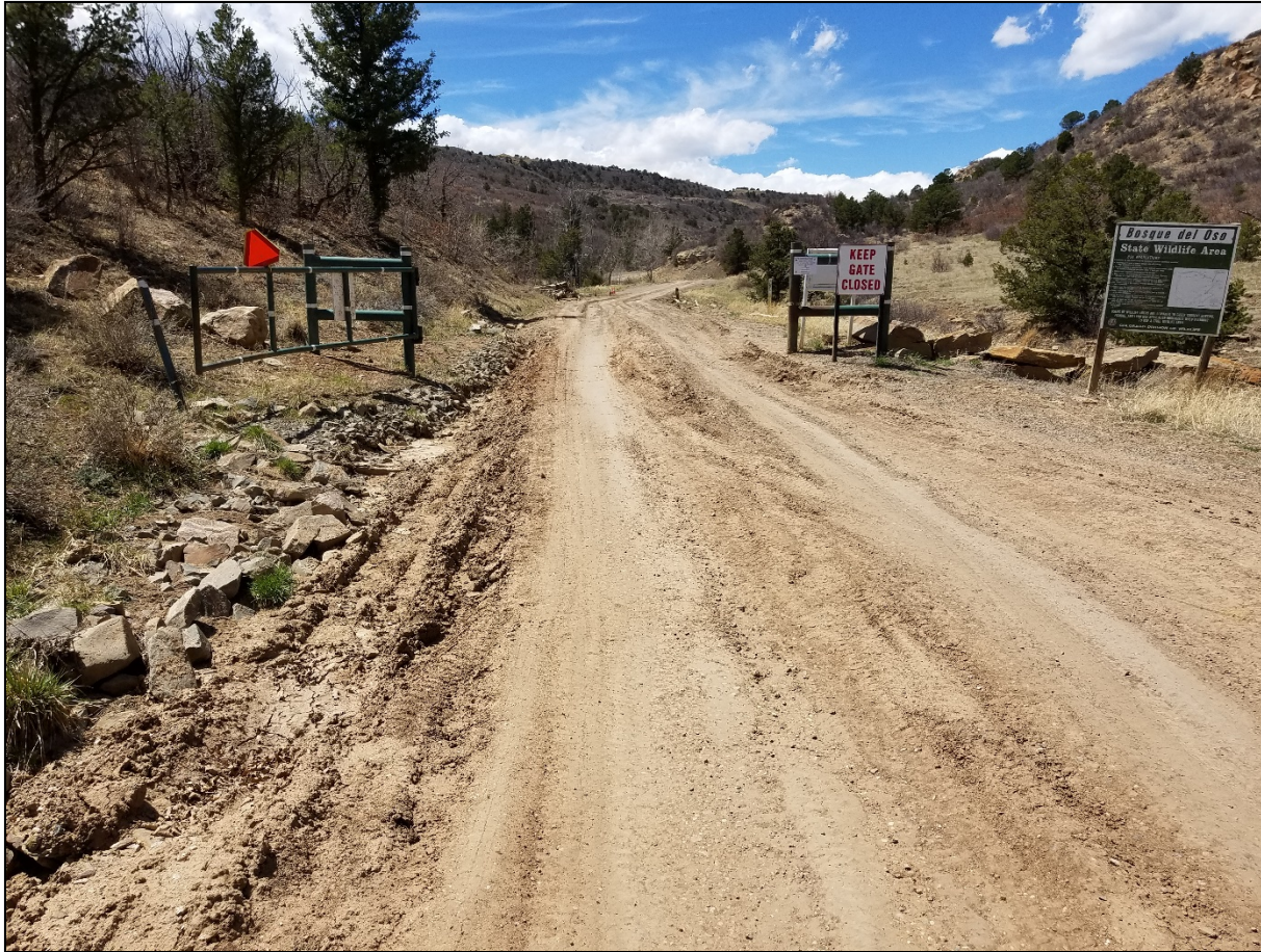
Photo 1. Facing northwest along the main road at the gate of Cherry canyon. Stormwater appears to have flowed down the road from a plugged culvert. There is vehicle rutting and erosion in this area.
