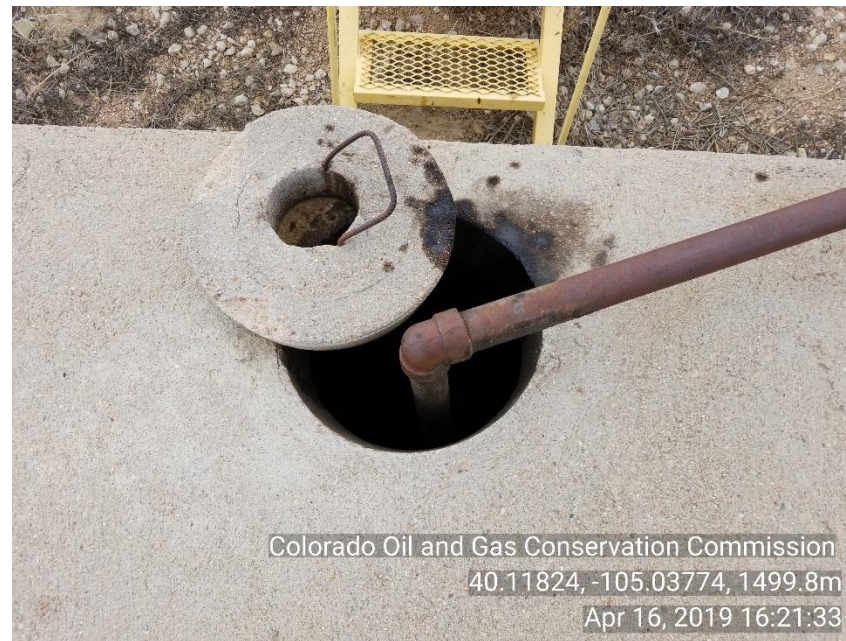
Photo 10 Wildlife issue no bird netting on top of produced water vault.
