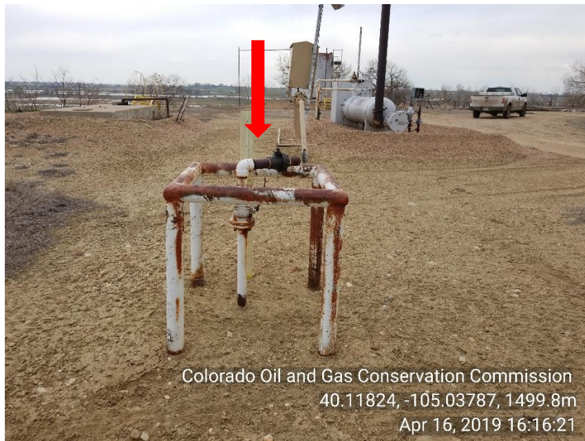
Photo 7 Unmarked unused and not LOTO Riser
