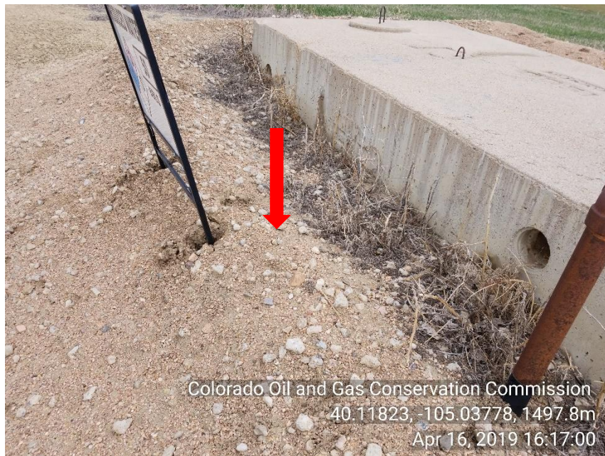
Photo 9 Inadequate berm around produced water tank.
