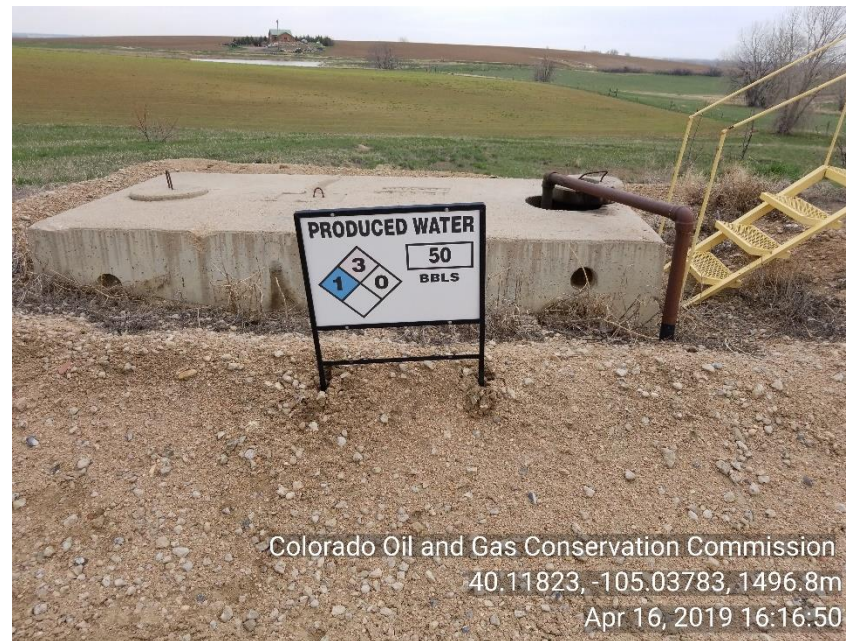
Photo 8 50 bbl produced water vault.
