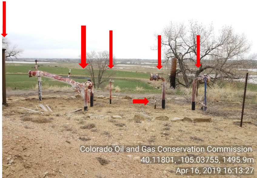
Photo 3 unmarked, unused risers
