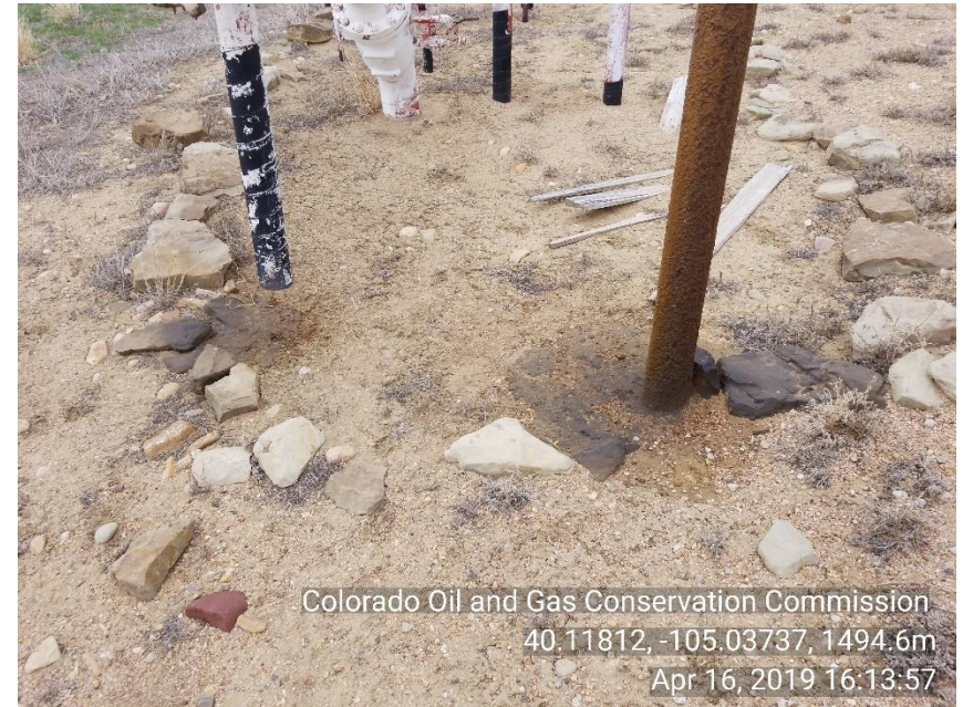
Photo 4 stained soil around risers next to pig launcher.
