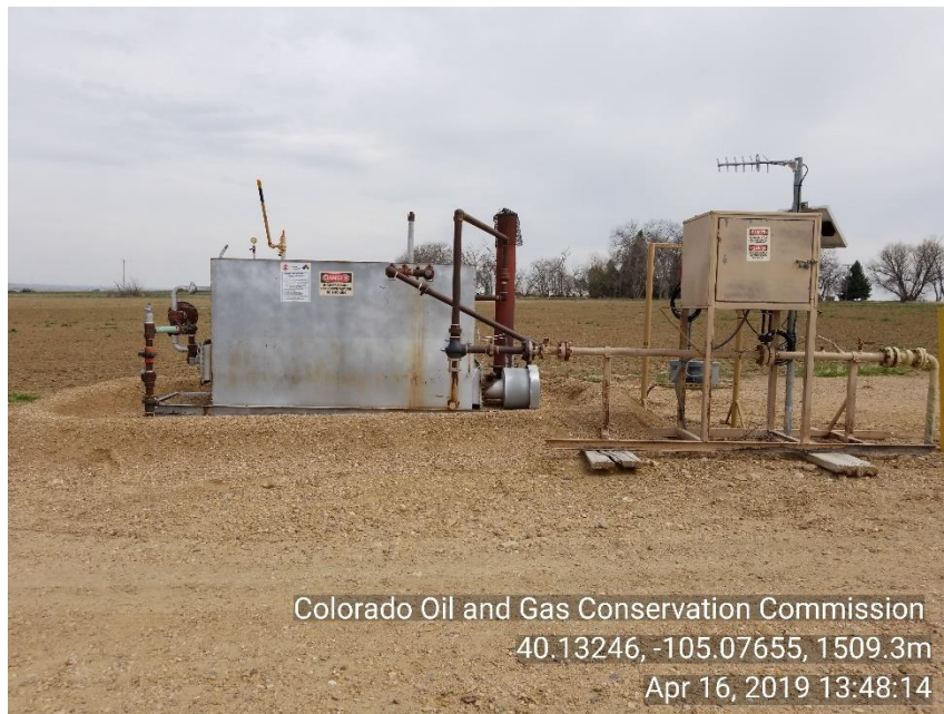
Photo 3 Sep and meter run
