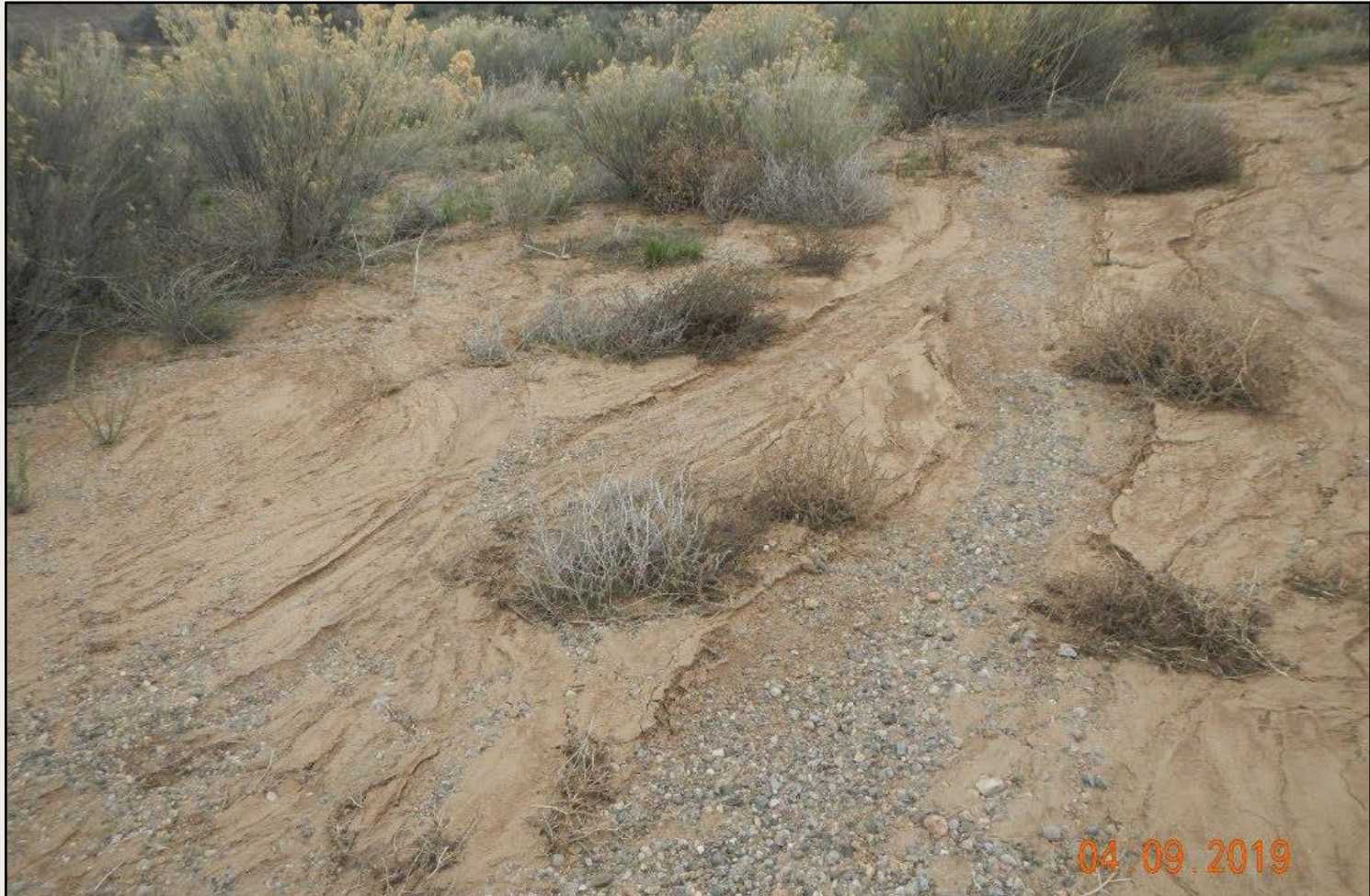
Photo 5. View of erosion within the northwestern portion of the project area, where stormwater flows from the access road appear to erode the road surface and carry sediment and debris downslope toward the northern drainage.
