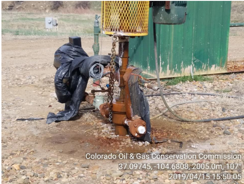
PHOTO 3: PACKING IS STILL LEAKING CAUSING APP. 3' ROUND AREA OF IMPACTED SOIL AROUND WELLHEAD
