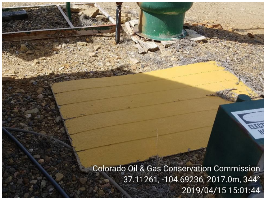
PHOTO 3: DEBREE ON LOCATION. A SECTION OF WELLHEAD HOUSE WALL HAS FALLEN OF AND IS ON THE GROUND NEAR SEPARATOR
