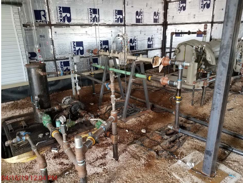
Photo 5 – Leaks within treater building
