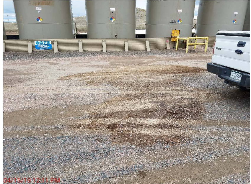
Photo 8 – Stained soil outside containment at crude oil loadout.
