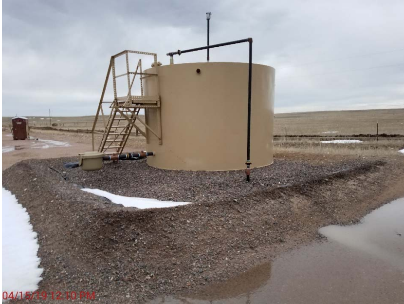
Photo 9 – Unlabeled AST – lacks NFPA, capacity and contents
