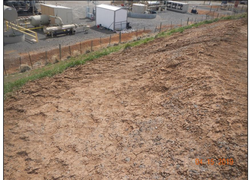
Erosion on side of tank moving soil down the hill
