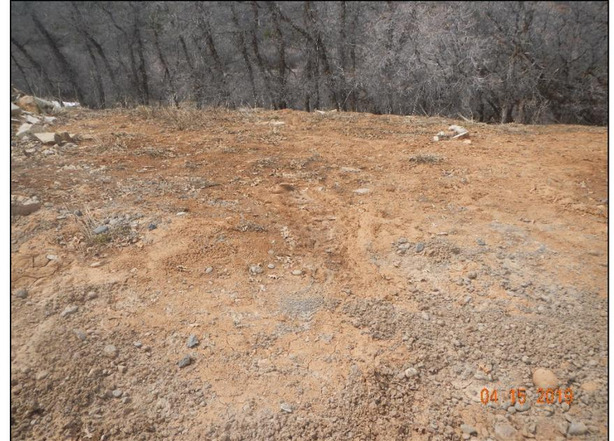
**Storm water moving sediment off location with no BMP**
