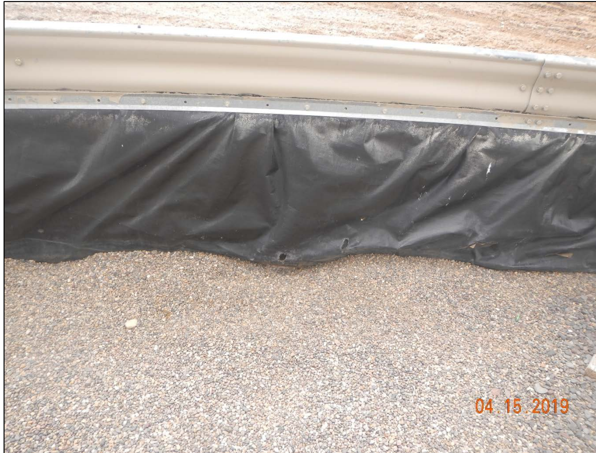
Holes in containment liner
