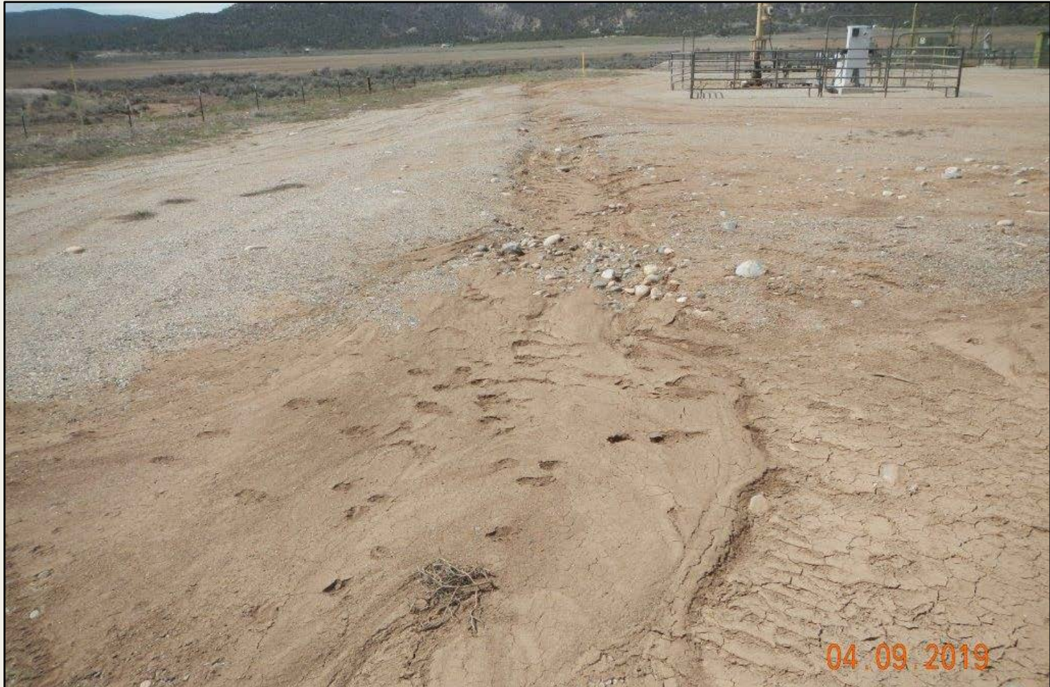
Photo 5. View of erosional channeling and sediment deposition within the southeastern portion of the working area.
