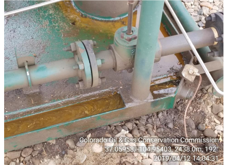
PHOTO 4: COMPRESSOR SKID CONTAINMENT IS FULL OF OILY WATER AND IS SPILLING OVER ON LOCATION IMPACTING SOIL ON NORTHWEST CORNER OF COMPRESSOR SKID.
