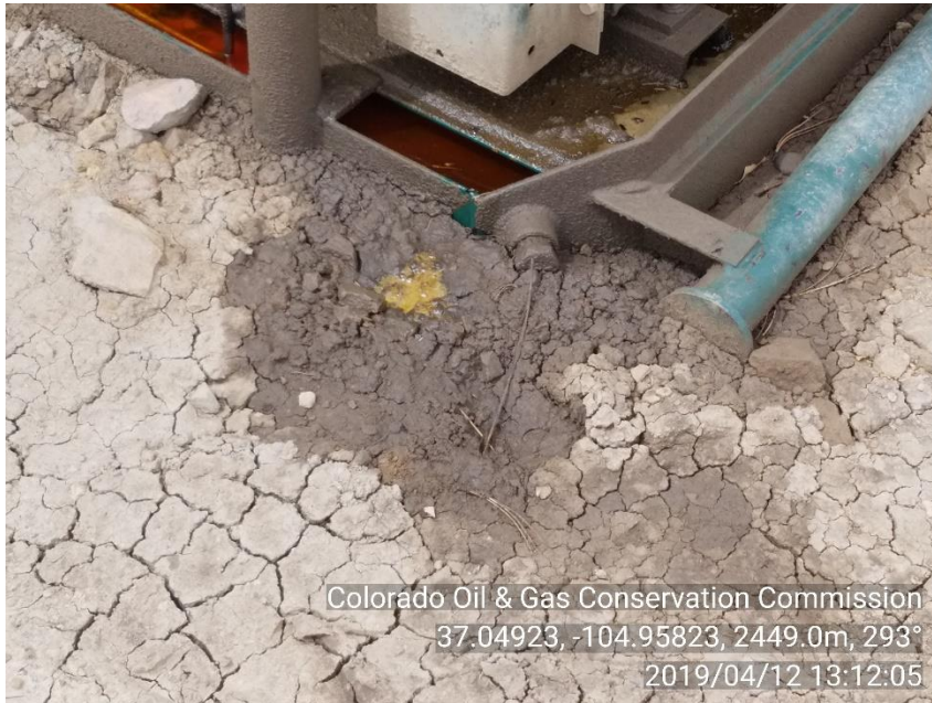
PHOTO 3: THERE IS APP. 2' AREA OF IMPACTED SOIL ON SOUTHEAST CORNER OF COMPRESSOR SKID NEAR SKID DRAIN PLUG.
