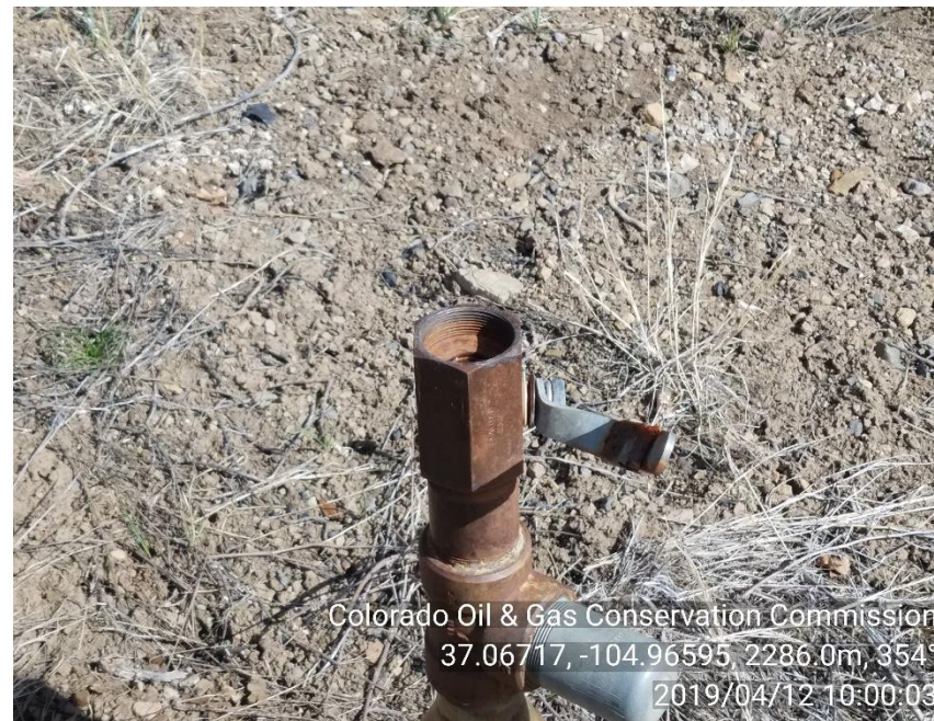
PHOTO 2: NO LO/TO ON WELLHEAD
